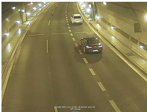
Figure 1: Activation of emergency escape lighting
