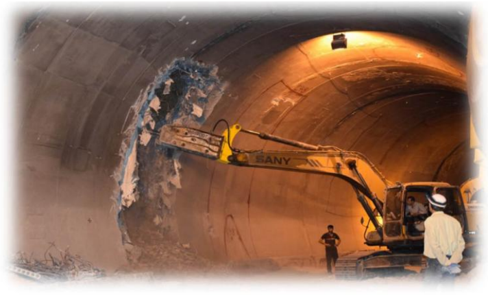
Figure 4: Tunnel integration and controlled demolition zones
