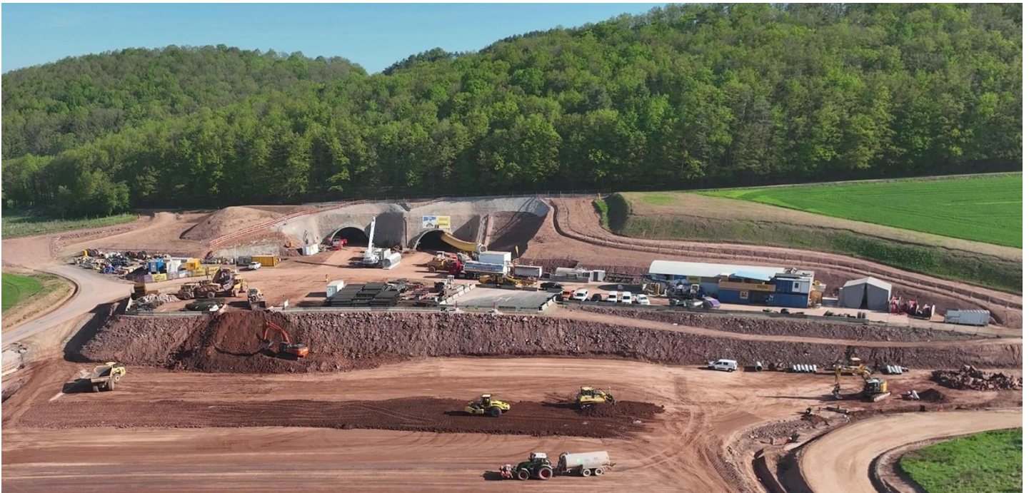
Figure 6: South portal including the construction site facilities.
