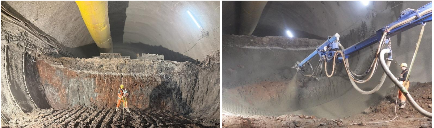
Figure 10: Bench excavation, Figure 11: Invert excavation with shotcrete application.
