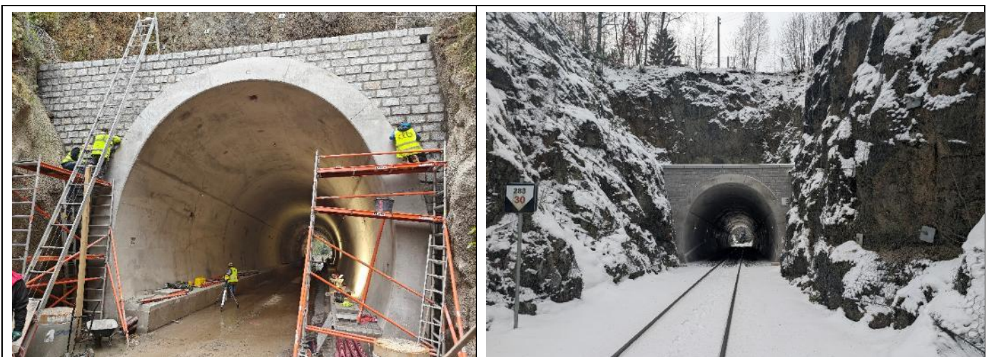
Fig. 15 Cladding of the new portal with natural stone and integration of the tunnel into the landscape
