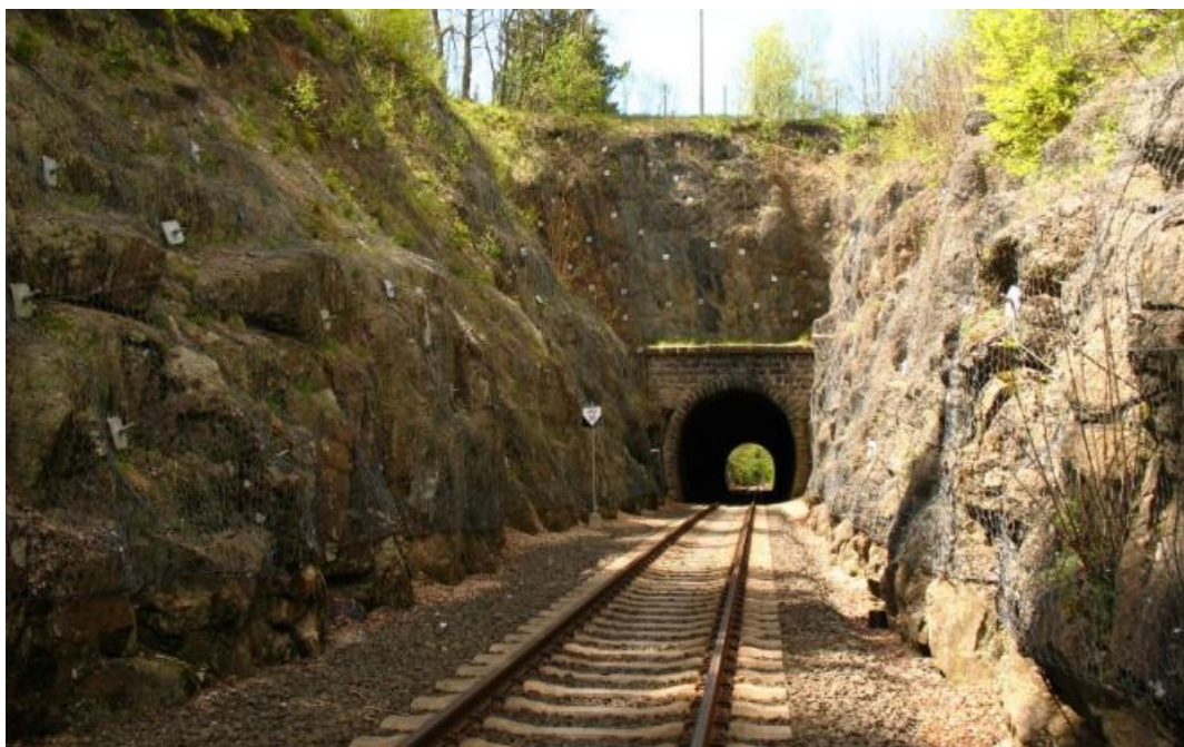
Fig. 13 Rock cut walls in front of the portal
