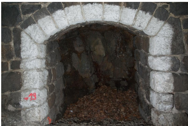
Figure 7 Rock in a rescue niche
