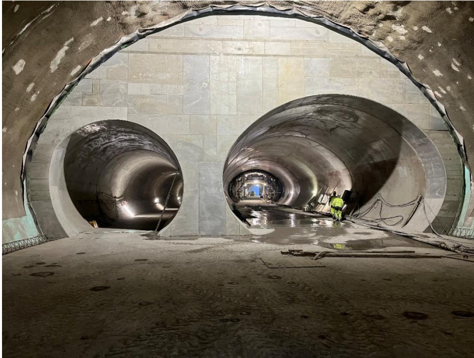
Figure 9 – Front wall of the junction to the lay-by tunnel
