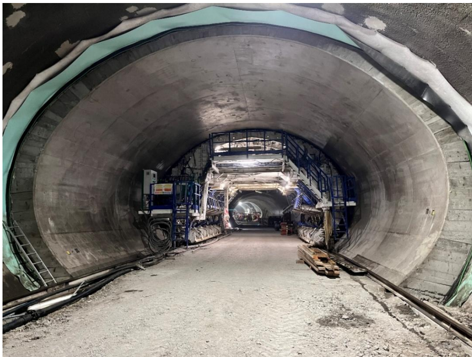
Figure 11 - Concrete pouring using a steel hydraulic formwork for a double-track tunnel
