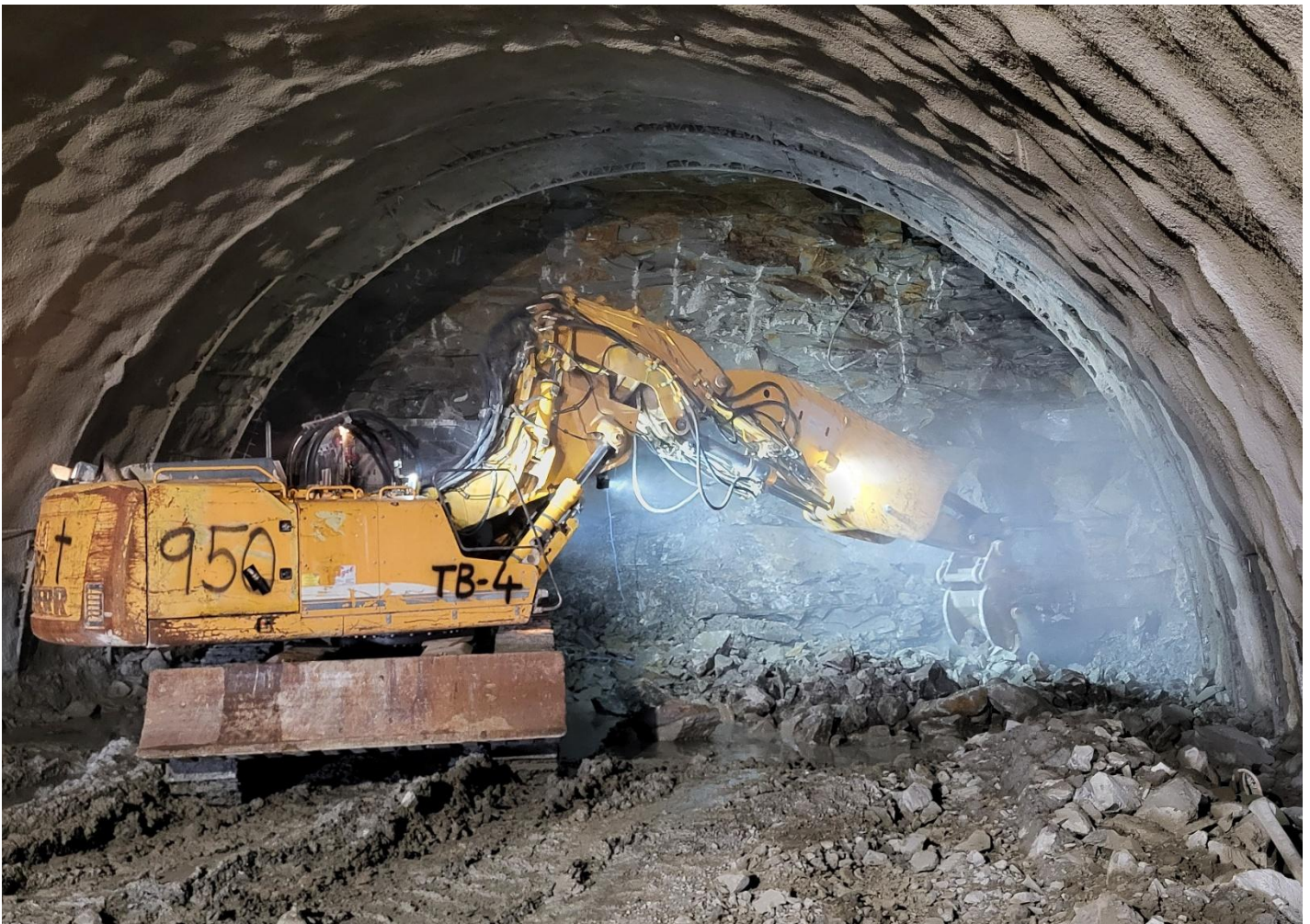
Figure 3: Rock excavation at LTT
