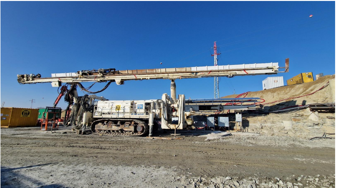
Figure 5: Equipment for installing micropile umbrellas
