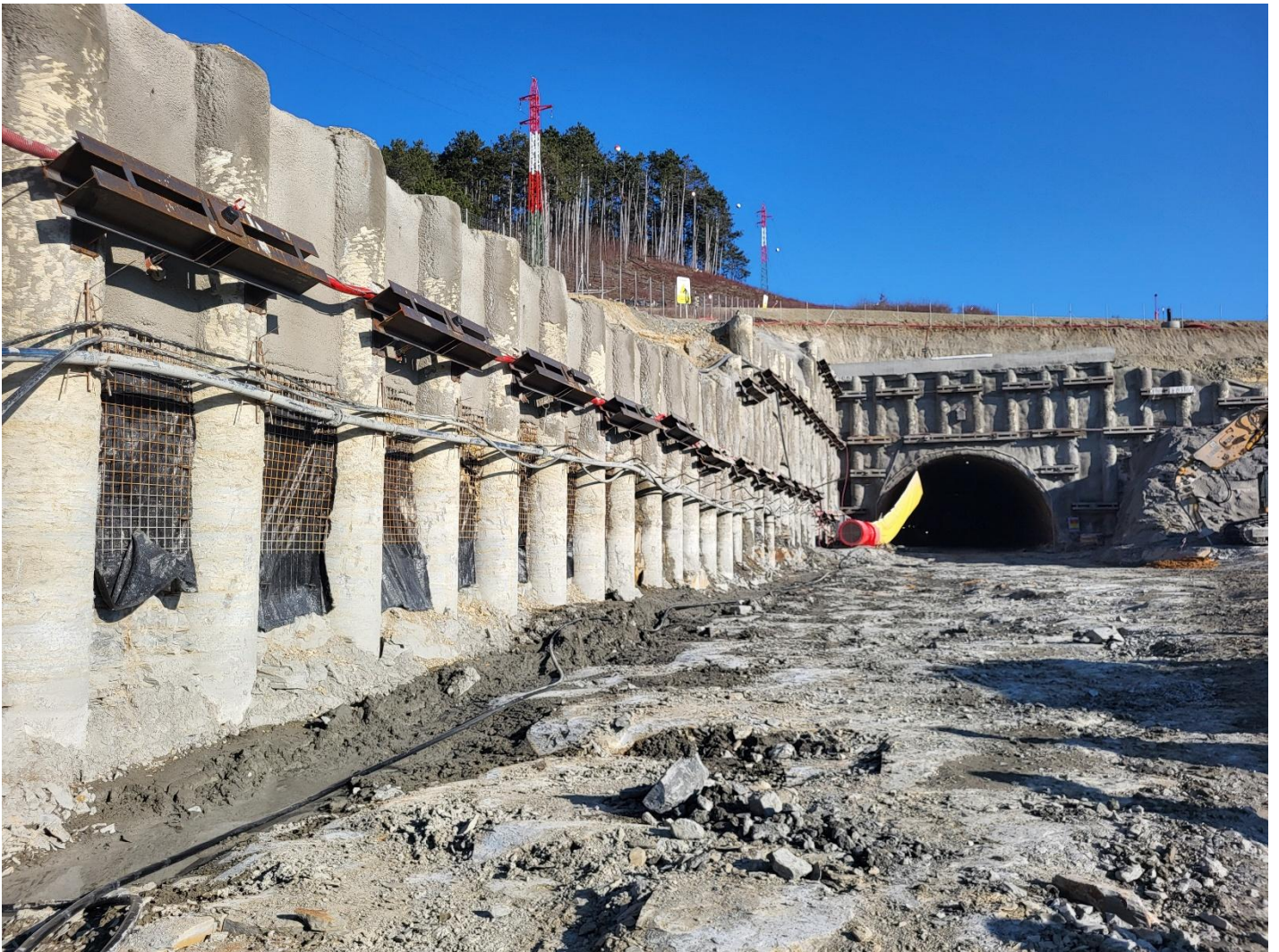
Figure 2: Support works for the construction pit at the western portal
