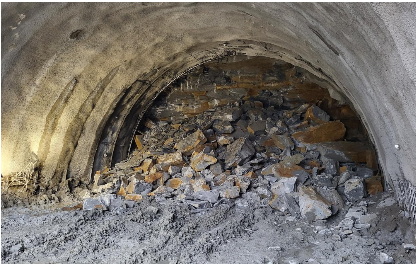
Figure 4: Rock Detachment in the LTT
