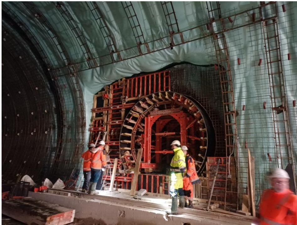
Figure: Preparation for concreting the cross passage block
