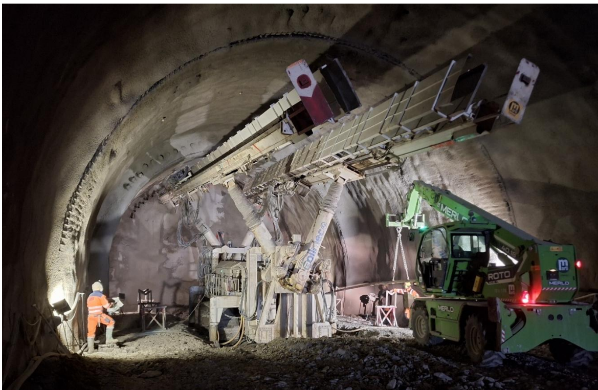
Figure 6: Soilmec ST 120 drilling rig installing pipe umbrella
