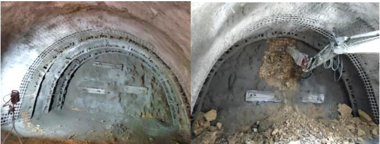
Figure 8 Tunnel face support and excavation sequence in the initial section
