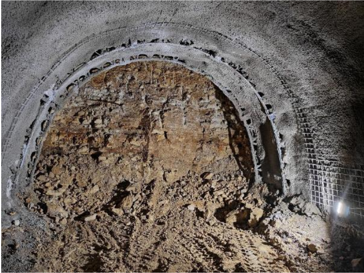
Figure 10 Top heading face consisting of slightly weathered marlstone (TM 66)
