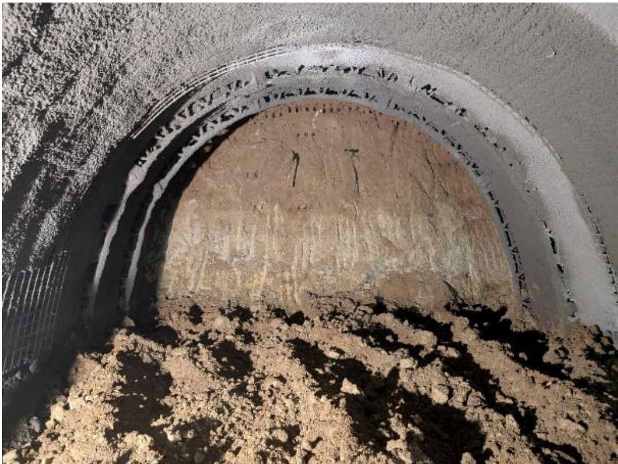
Figure 11 Top heading face consisting of clayey soil (TM 264)
