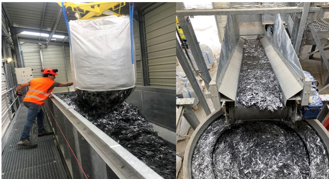
Figure 3: Dosing equipment installation specially design for glued fibre.
