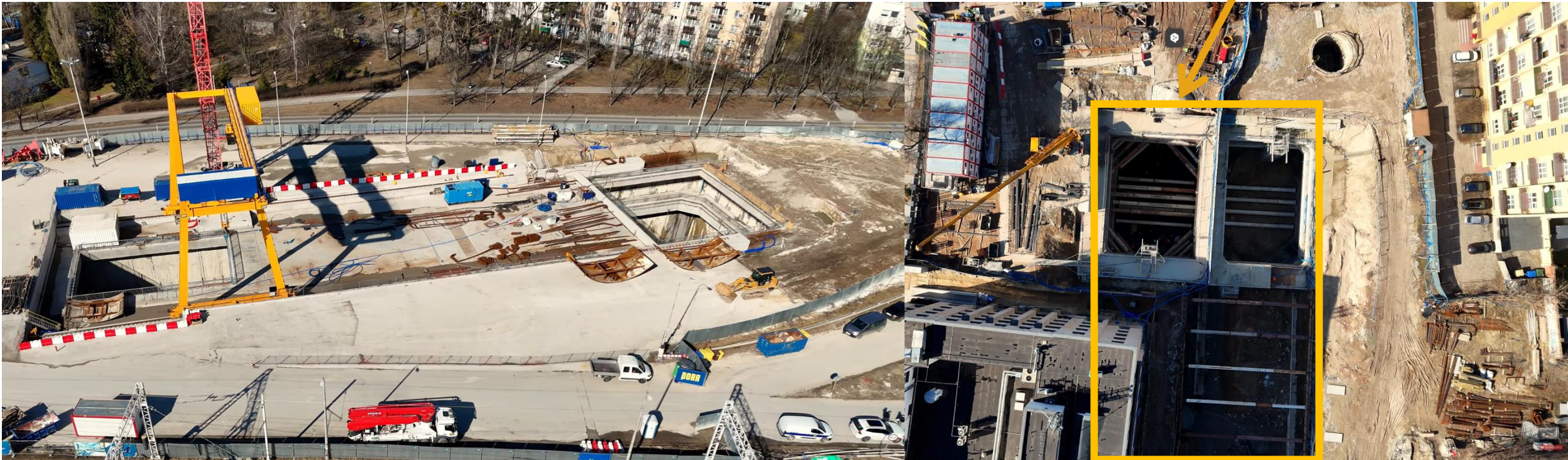
Starting shaft „Retkinia” Works for TBM assembly and launching in progress
