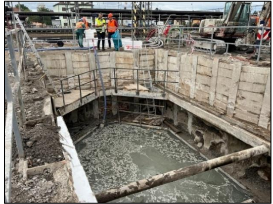
Figure 6: Flooding the shaft to prevent bottom break through.
