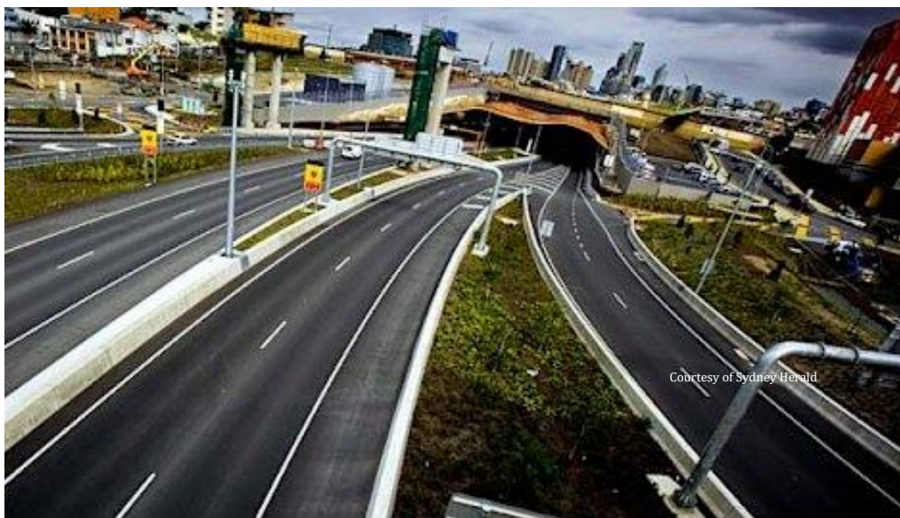
Figure 5 – Clem Jones Tunnel, Brisbane, Australia
