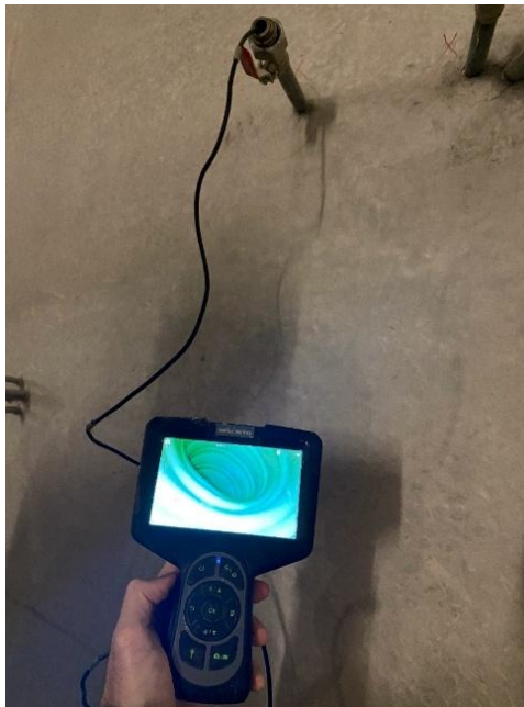
Figure 7: Conducting a video inspection through a grouting packer (source: Camós-Andreu)
