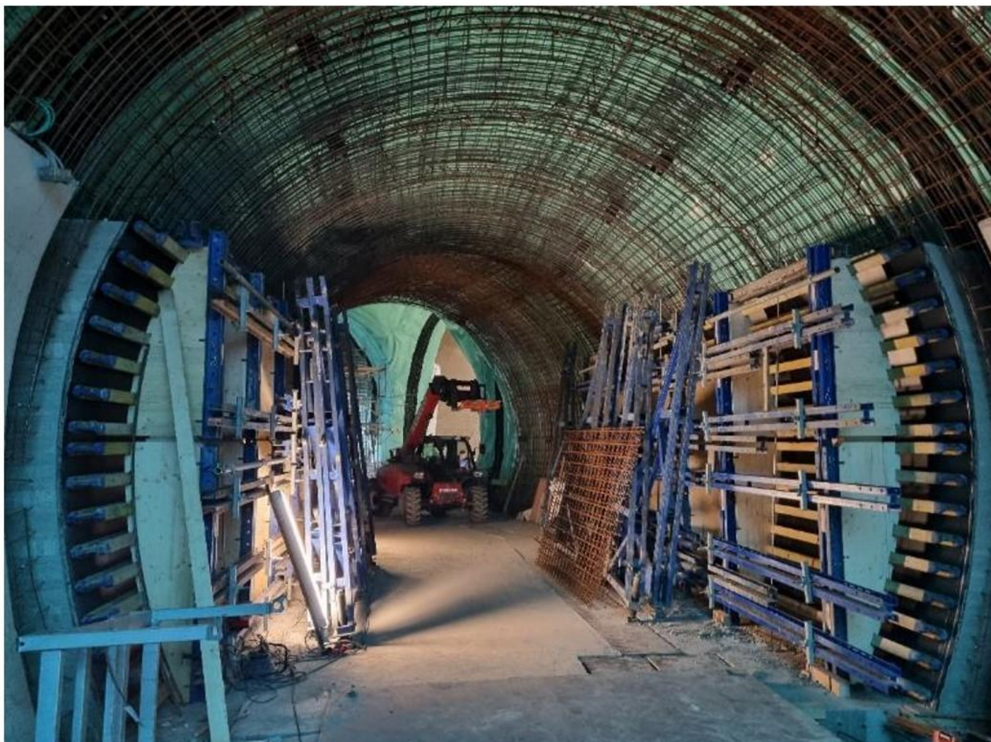
Figure 10: Formwork elements for secondary lining
