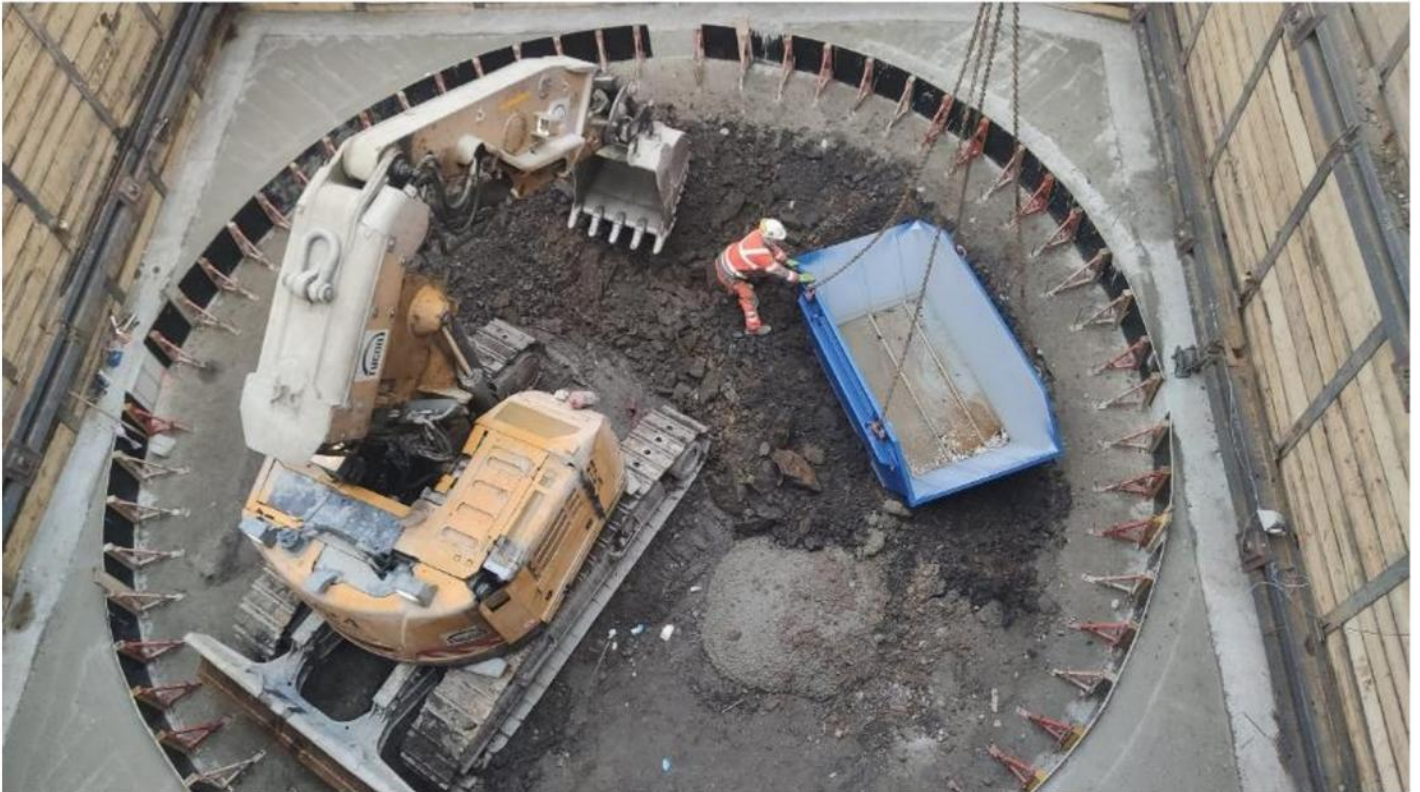
Figure 2: Extraction of rubble using a crane and a container
