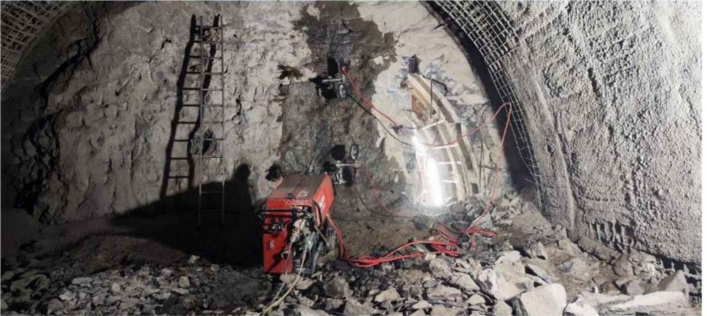
Figure 4: Cutting the reinforced concrete front wall with a diamond wire
