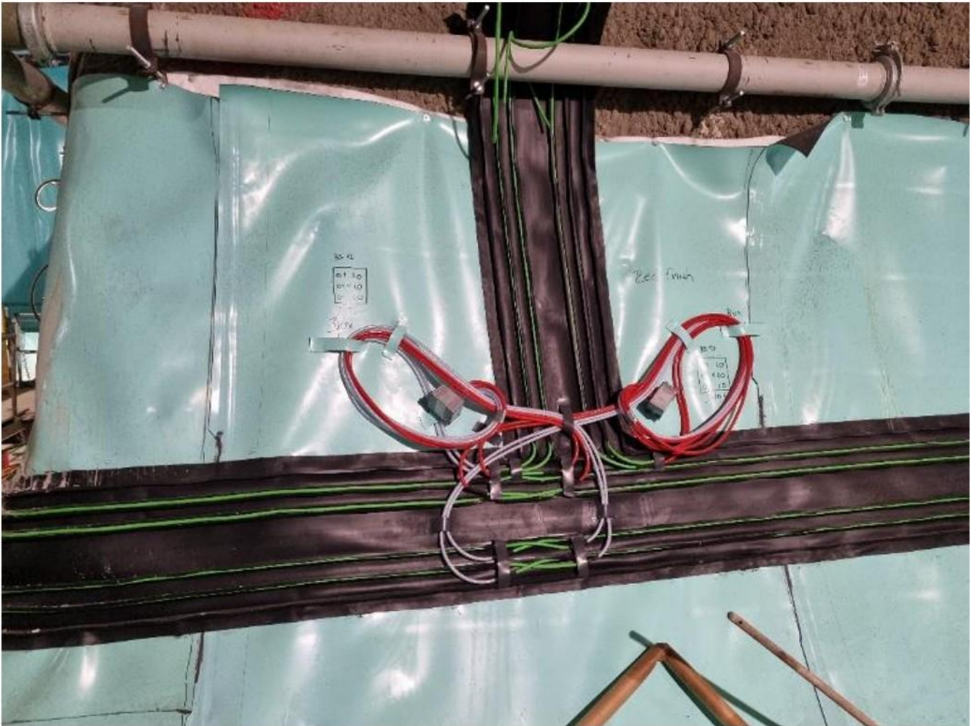
Figure 8: External joint strip with injection hoses
