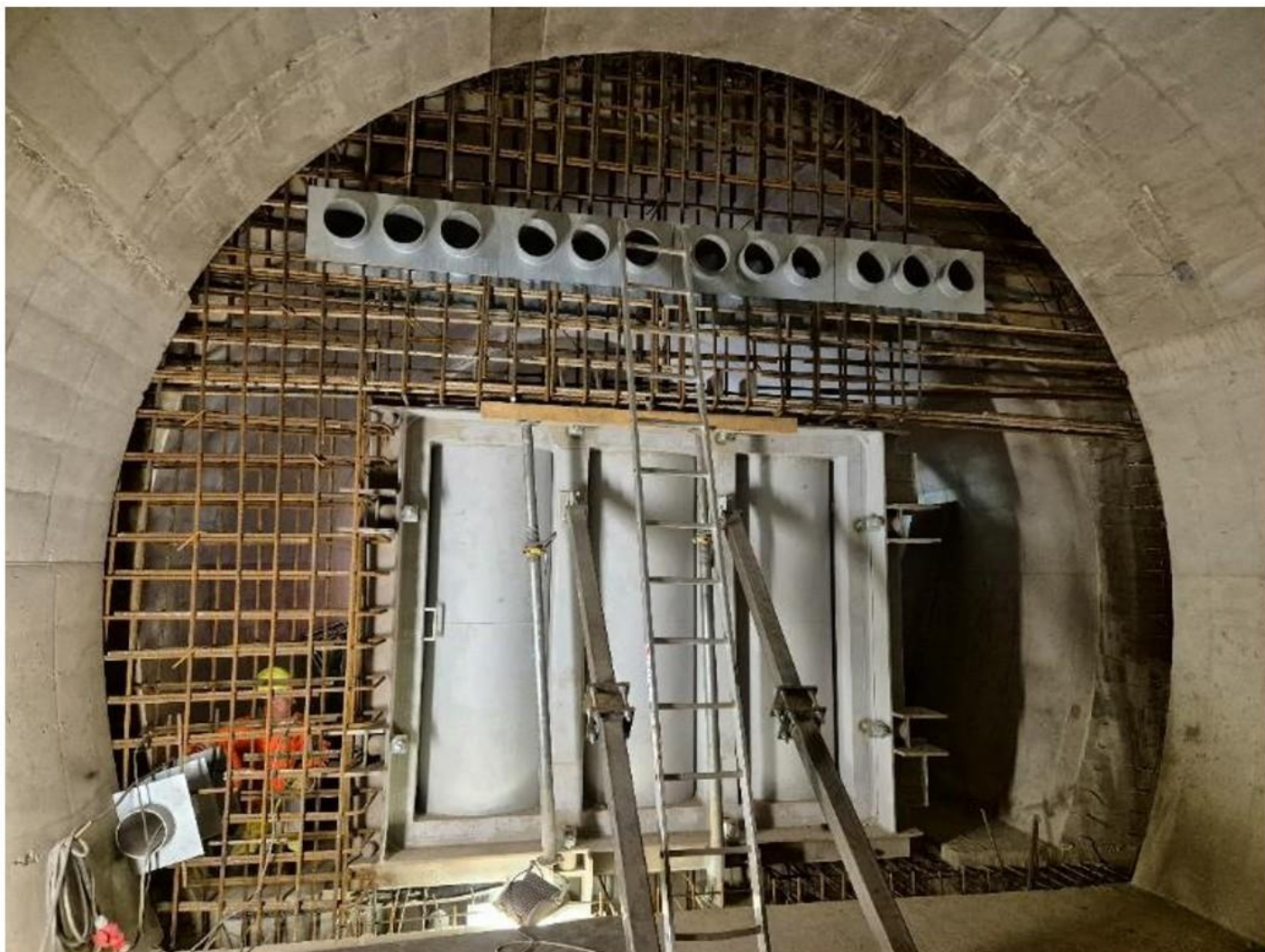
Figure 9: Preparation for concreting the pressure seal
