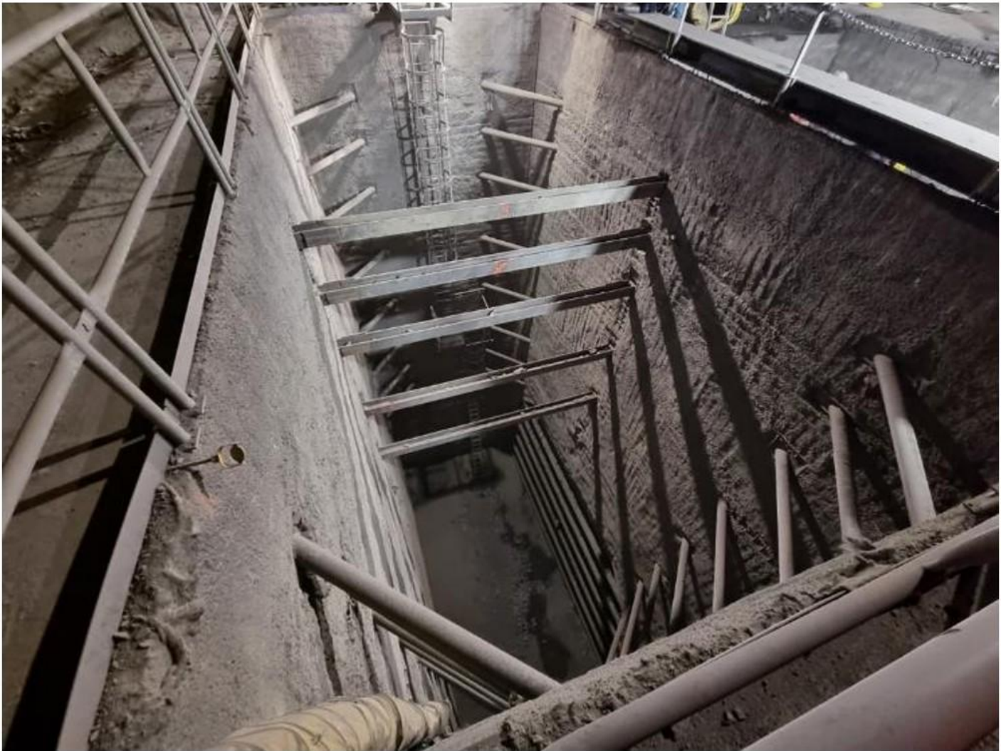
Figure 3: Lift shaft Š2.2
