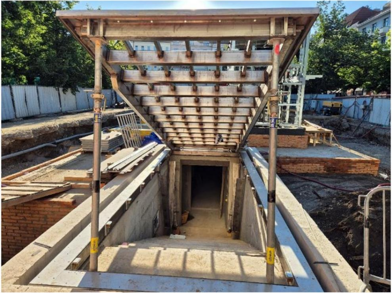
Figure 11: Escape hatch after installation
