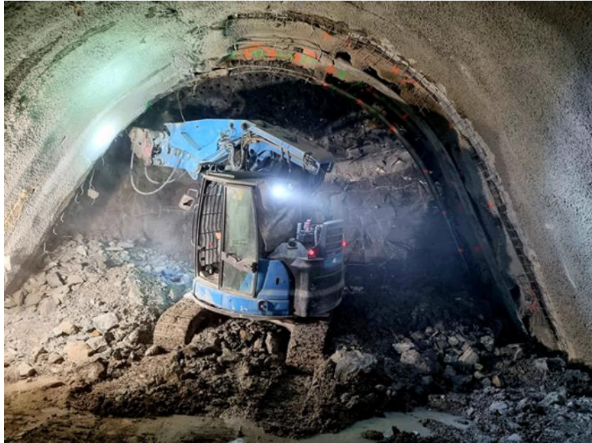
Fig. 3: Excavation of the base gallery
