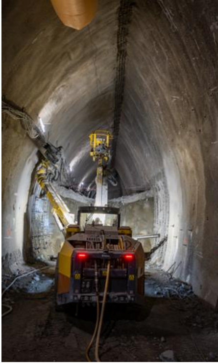
Fig. 6: Bench I excavation
