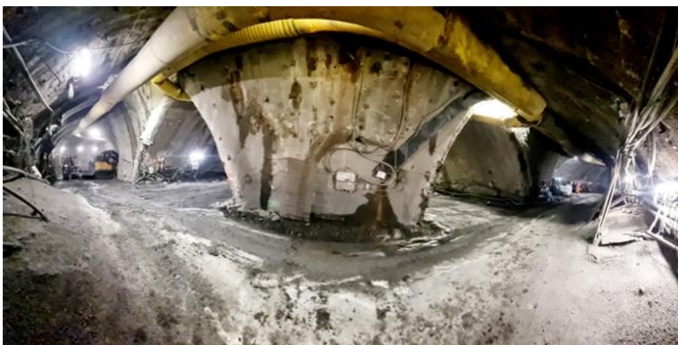
Fig. 5: Excavation of side profiles
