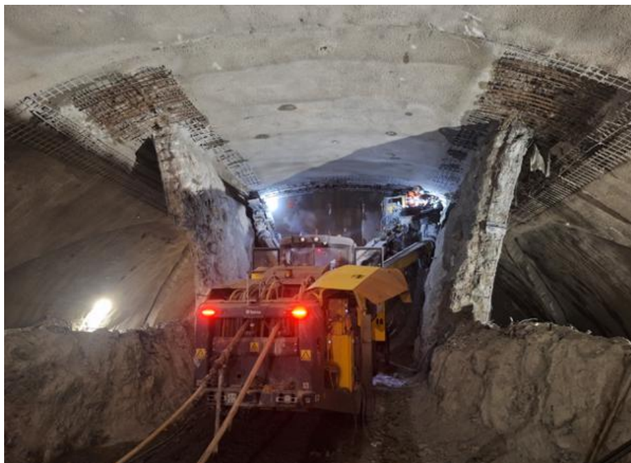
Fig. 9: Middle profile top heading excavation
