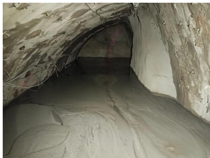
Fig. 8: Filling the transfer section with TERRAFLOW infill concrete
