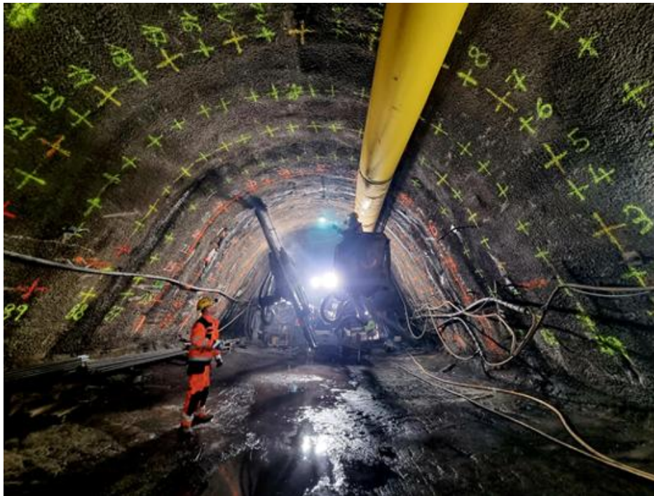
Fig. 4: Injections from the toe tunnel
