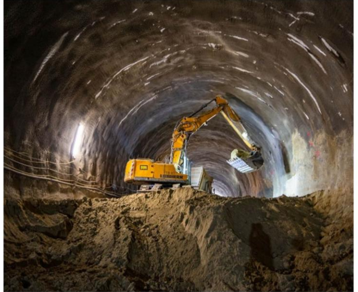
Figure 6: Excavation of the invert
