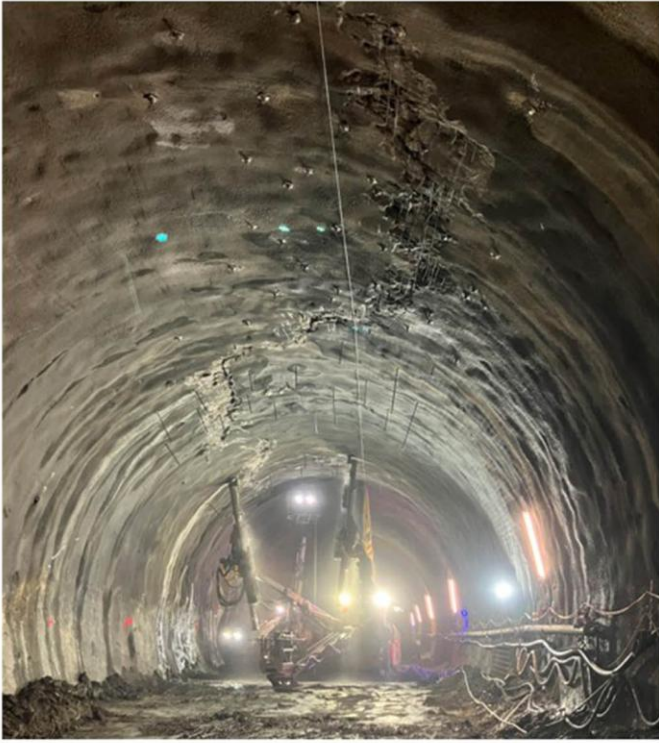
Figure 9: Repair work after the crack
