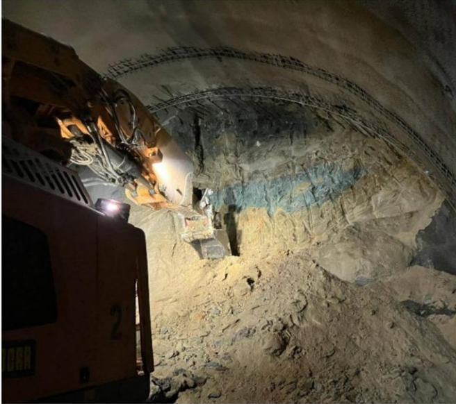
Figure 5: Top heading excavation in sand and clay
