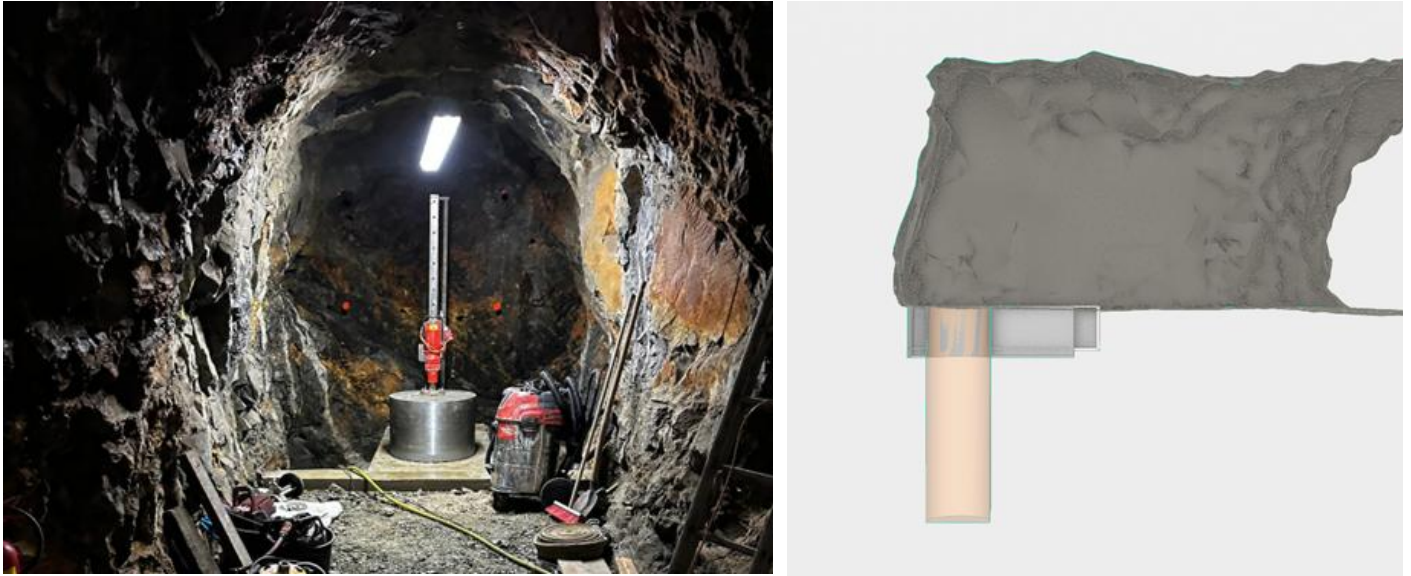
Figure 6 – On the left is a photo taken during the drilling of a borehole for the INTES project experiment, and on the right is a conceptual design of the experiment, where waste materials from foundries will be tested for energy storage..
