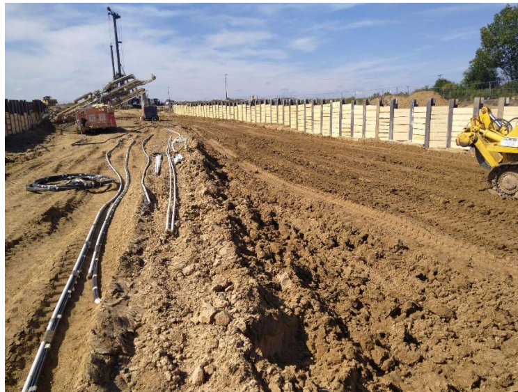
Figure 4: Pile shoring in the initial construction phase
