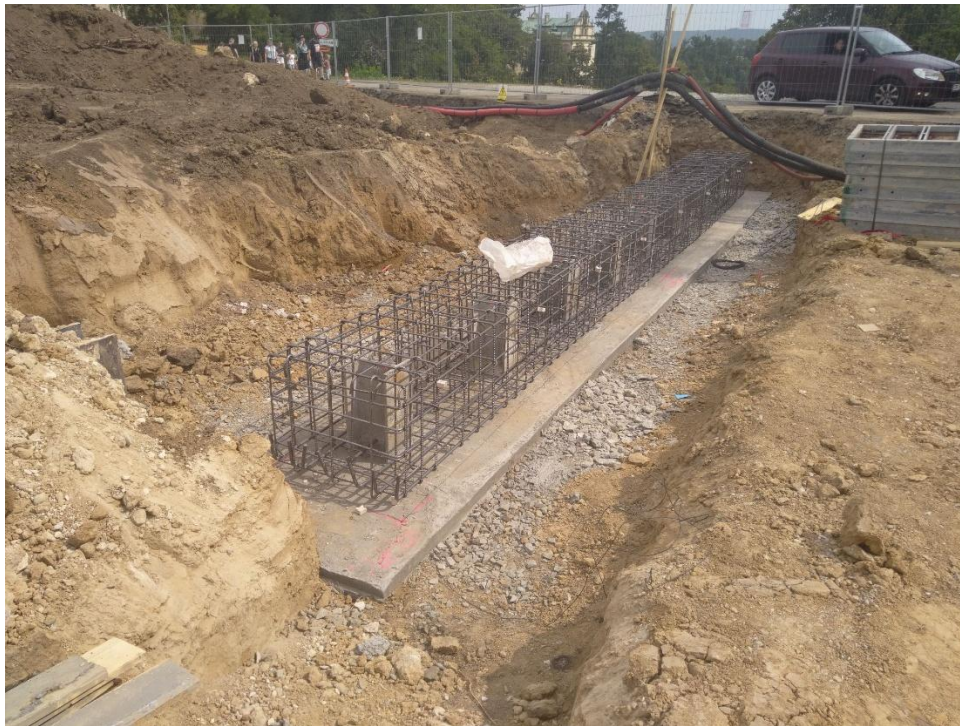
Figure 5: Temporary bridge foundation during construction
