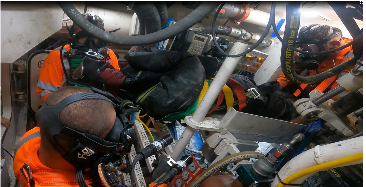
Figure 4: Rescue exercise “evacuation from excavation chamber”
