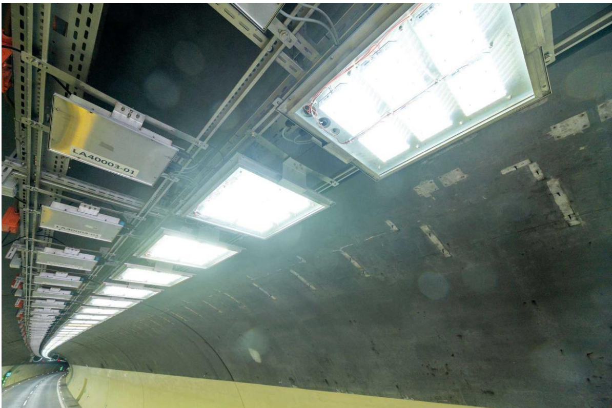
Figure 3: Completed new LED lighting in the entrance adaptation zone
