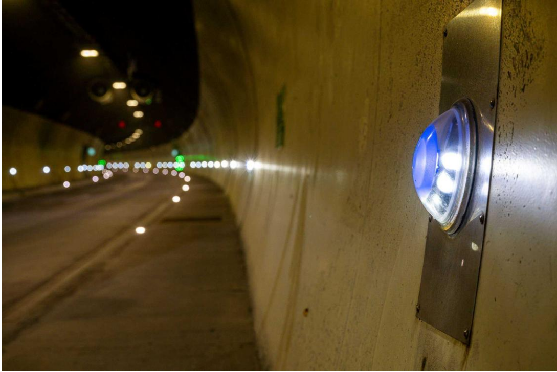
Figure 4: Emergency lighting luminaire with positioning blue LED
