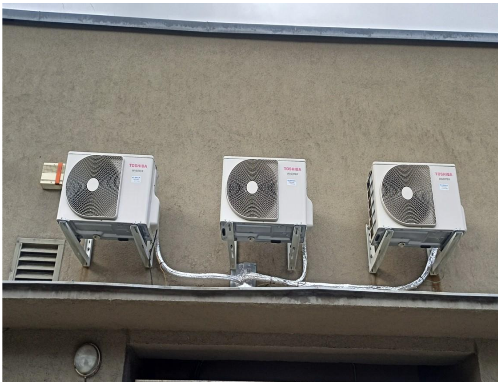
Figure 14: Newly installed PTO cooling
