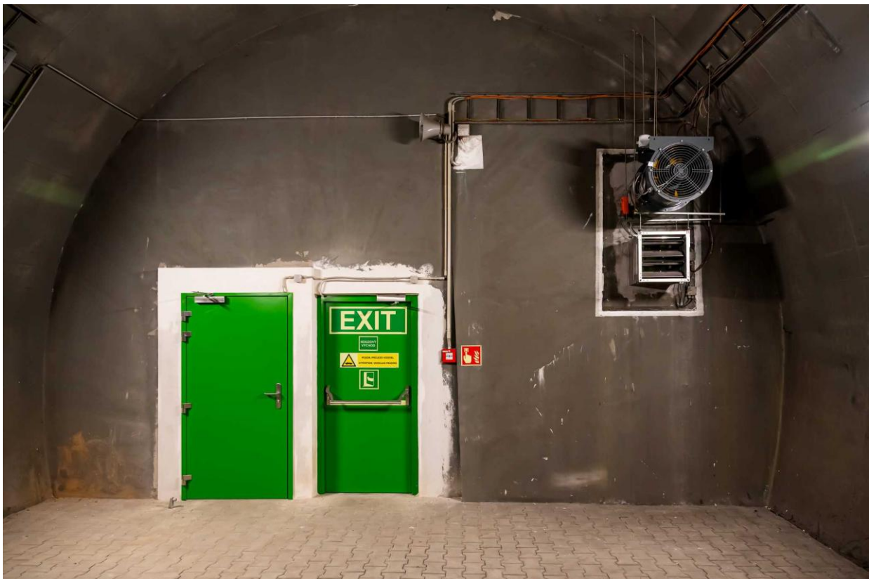
Figure 13: Newly installed cross-passage ventilation equipment
