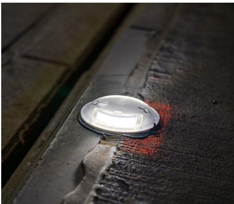
Figure 5: Inductive guidance lighting – detail of the luminaire
