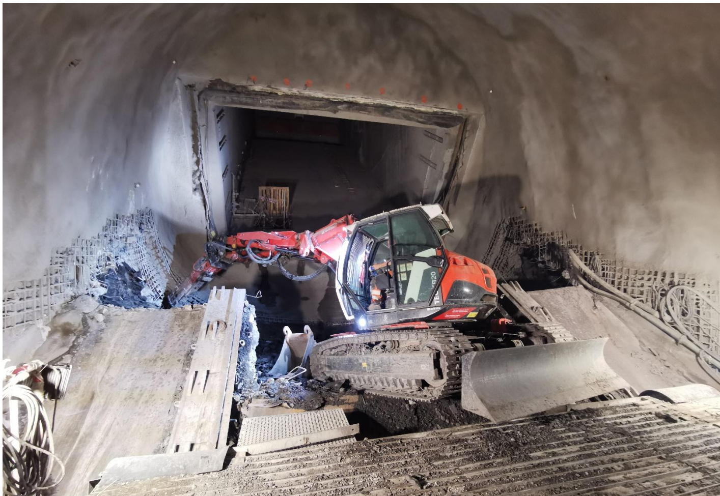
„Fig. 4b – Excavation of the lower vault of the escalator tunnel“
