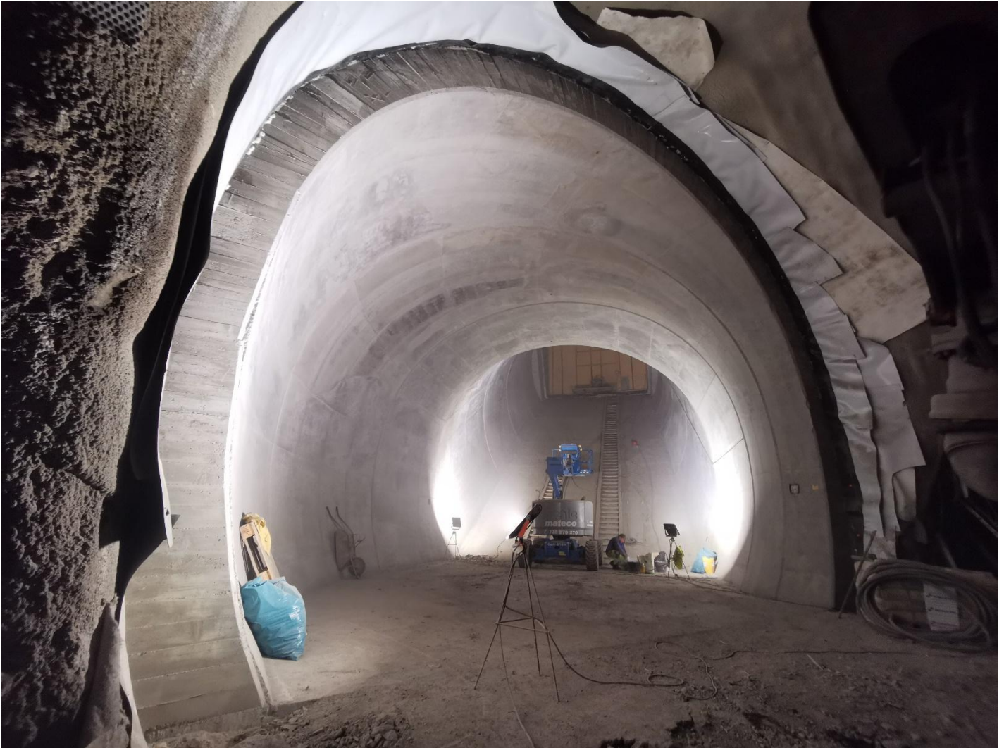
“Fig. 7 – Fully completed secondary lining”
