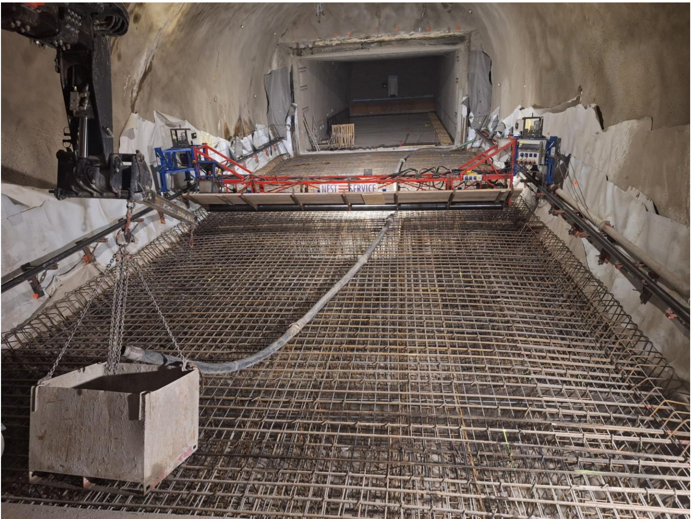
„Fig. 5 – Finisher for concreting the invert (bottom arch) “
