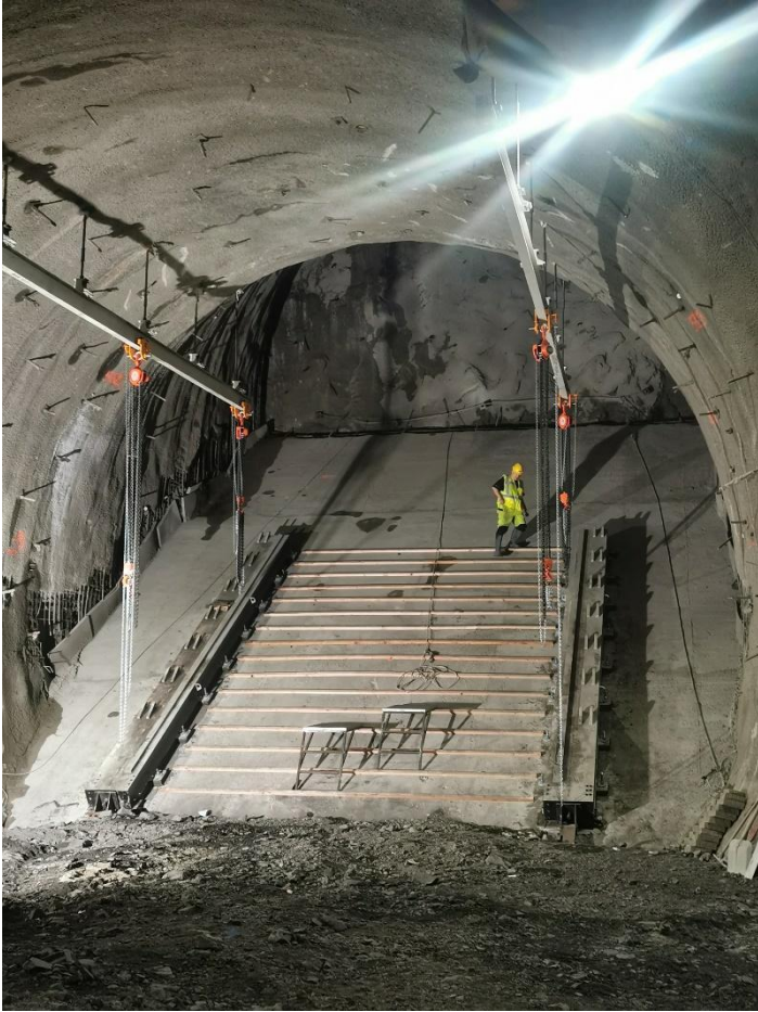
"Fig. 3 – Suspended rail system for platform installation"
