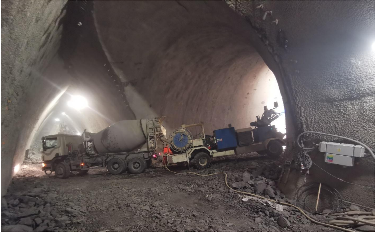
“Fig. 2 – Commencement of excavation of the transfer corridor top heading”
