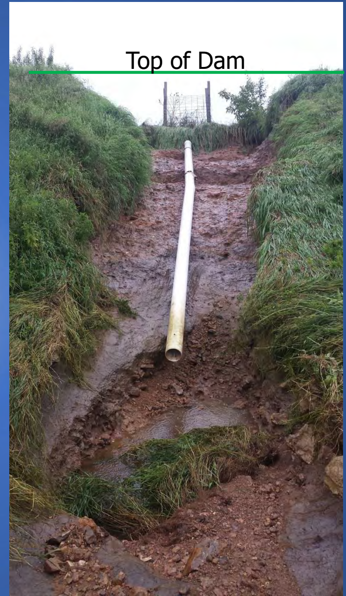
Grade Stabilization Structure
