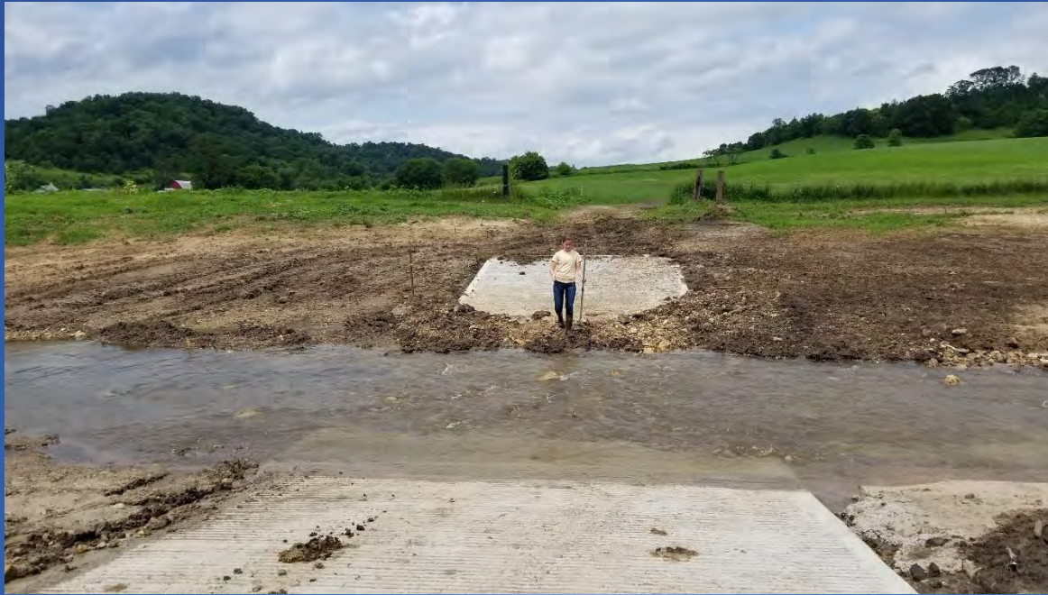
July 1 st – Concrete Stream Crossing
