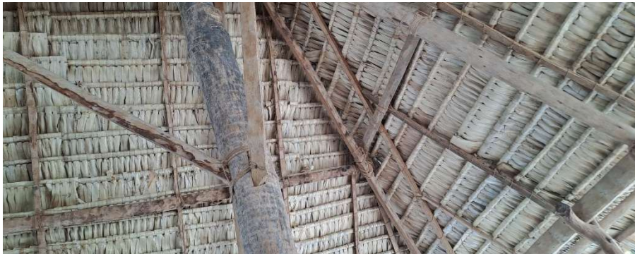
Figure 5: Intricate weaving of bamboo in the ceiling of a Maneaba in Kiribati. Source: Author
