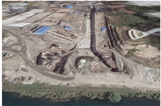
Figure 3. Construction of Agua Clara Locks, April 2011. ©Google Earth.
