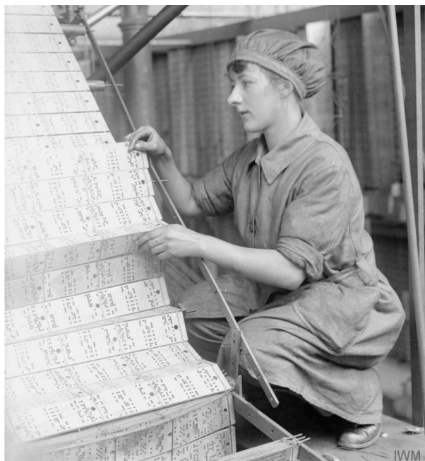
Fig 2. A female worker changing jacquard cards in a lace making machine. Lewis, George P. (Photographer), 1918. [ https://commons.wikimedia.org/wiki/File:The_Employment_of_Women_in_Britain_1914-1918_Q28124.jpg ]
