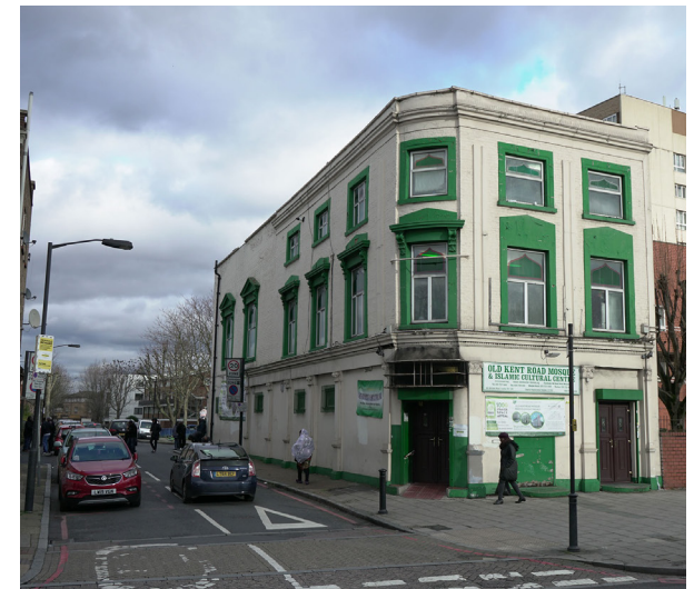
Fig.1 Outside view of Old Kent Road Mosque prior to demolition.
