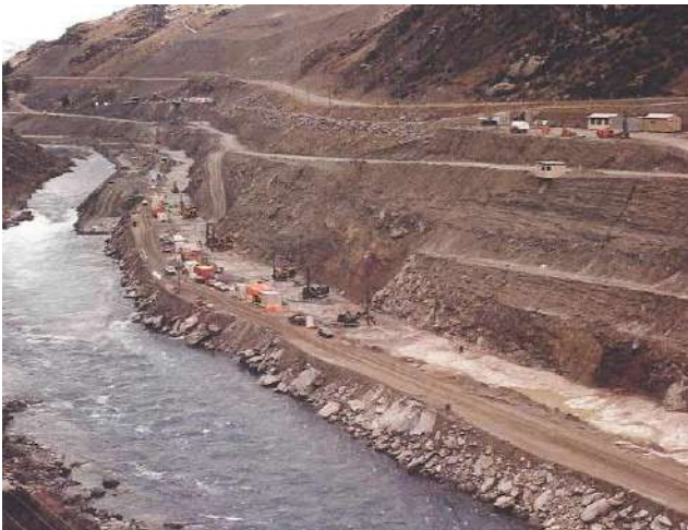
Figure 34. Grout curtain under construction at Brewery Creek (Clyde Power Project, unpublished).
