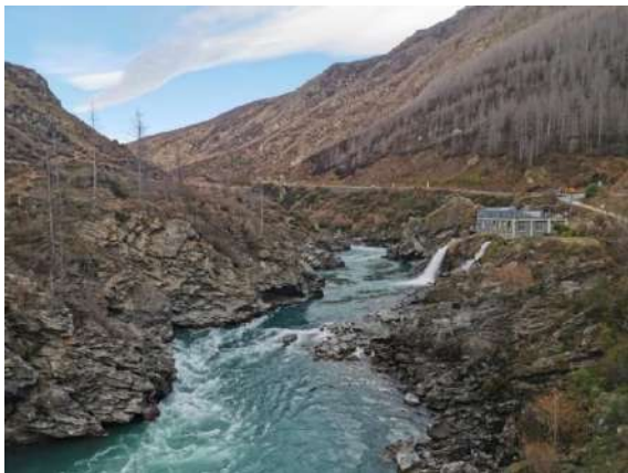
Figure 14. Looking upstream to the Roaring Meg Power Station.
