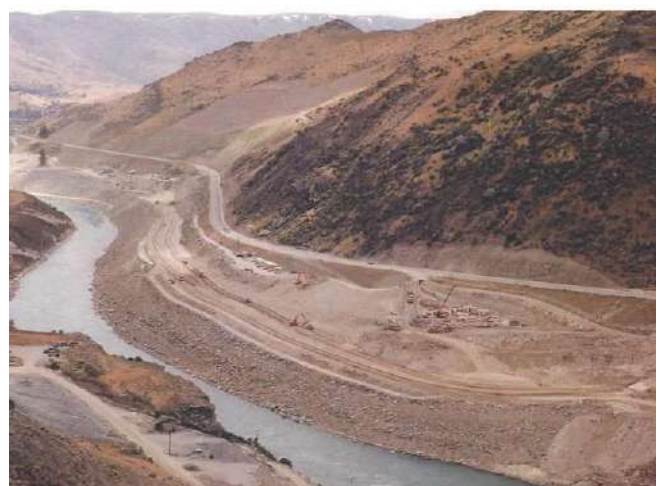
Figure 35. Constructing toe buttress, Brewery Creek slide (Clyde Power Project, unpublished).
