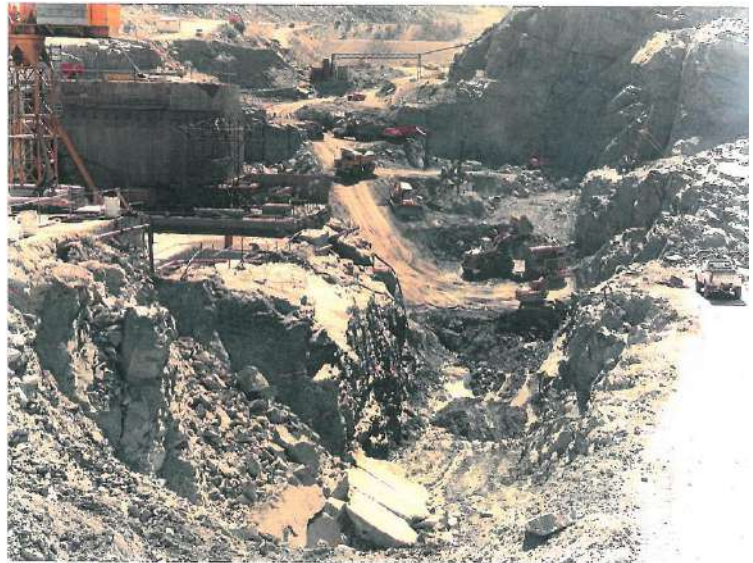
Figure 27. Looking upstream along the River Channel Fault remedial excavation (Thomson, 1993).
