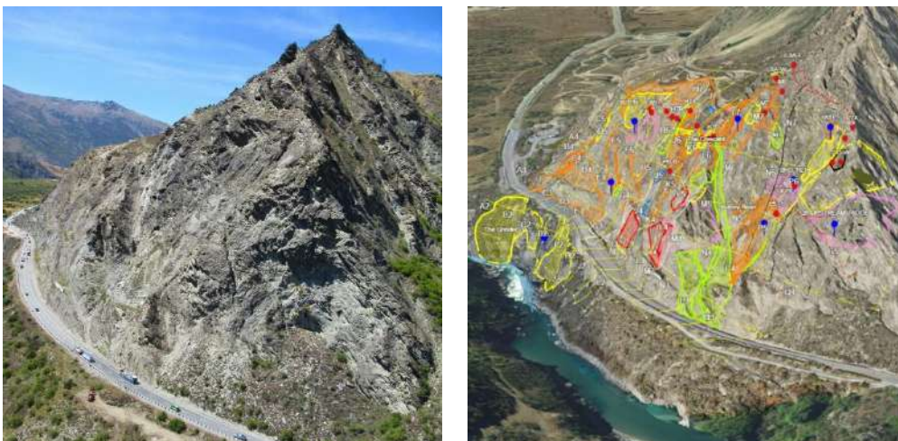
Figure 13. Drone image of Nevis Bluff and the digital twin developed to identify and manage risk (WSP, 2025).
