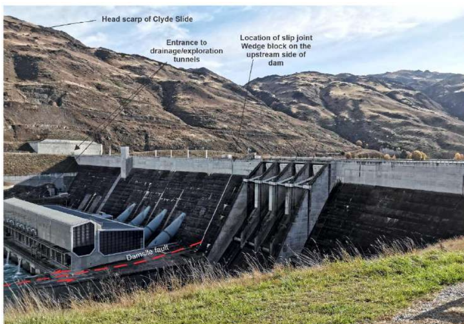
Figure 24. Clyde Dam with the Clyde Slide in the background. Photograph taken in May 2019.
