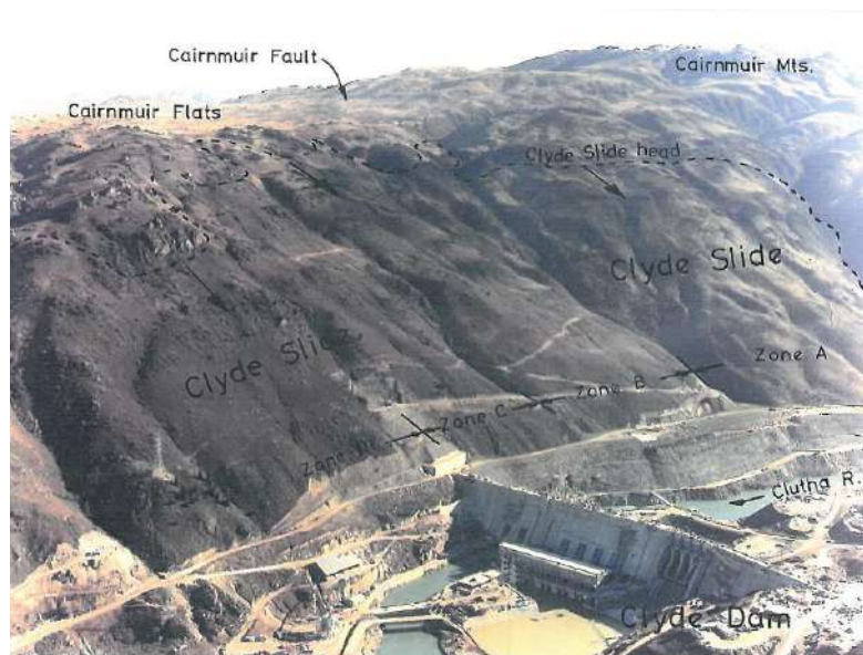
Figure 28. Clyde Slide taken during construction phase in 1989 (Thomson, 1993).
