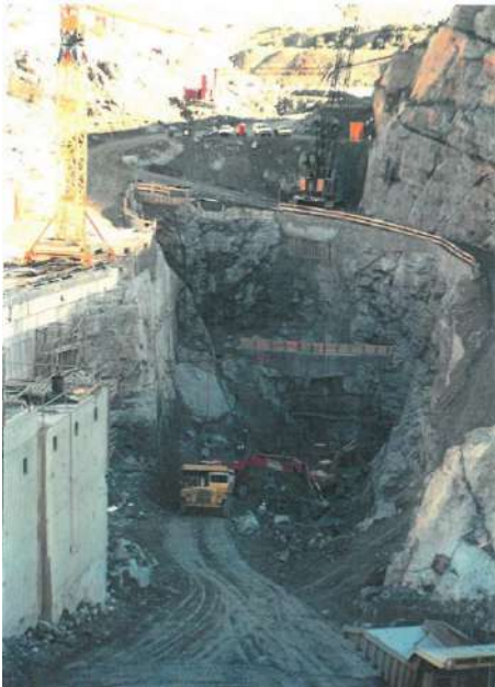
Figure 26. Looking upstream along the River Channel Fault, the orange colour excavator is located close to the River Channel Fault cut-off shaft (Thomson, 1993).
