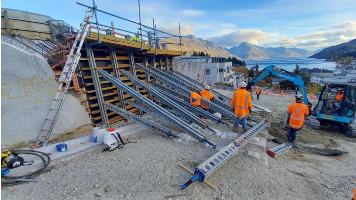
Figure 6. Propping for Beetham St tie-in in-situ facing pour.
