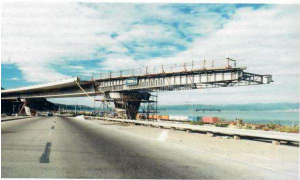
Southbound flyover bridge being pushed over the Hutt Road.
