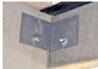
(b) Concrete to concrete connection
