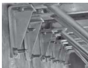
Figure 10. Chemical anchoring with anchor studs
