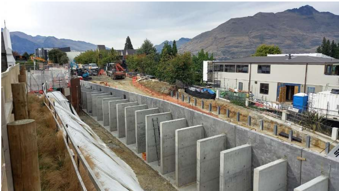
Figure 4. St Josephs Wall counterforts prior to backfill.
