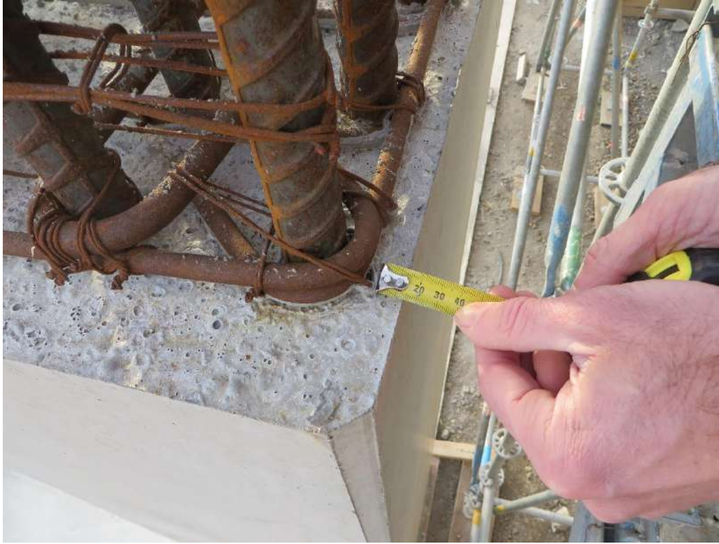
Column with less than 30mm minimum cover in marine environment
