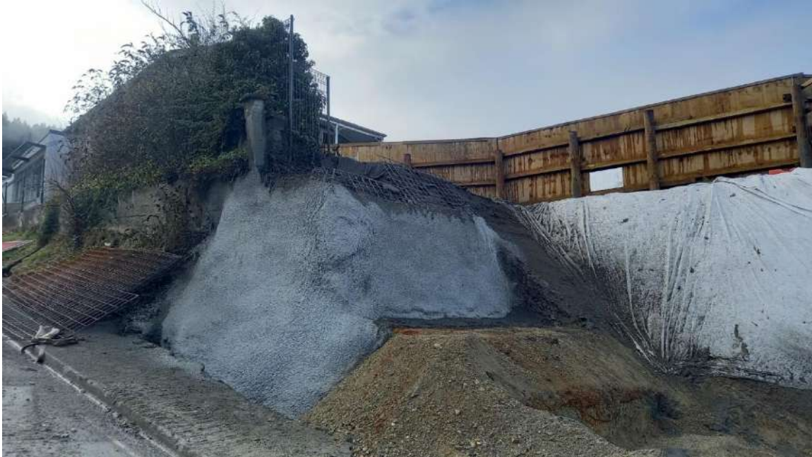
Figure 5. Shotcrete stabilisation of the Beetham Street tie-in.
