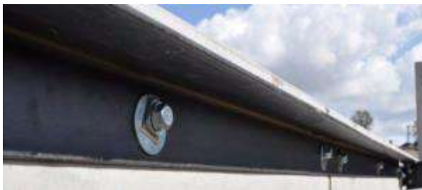
(a) Steel to concrete connection.
