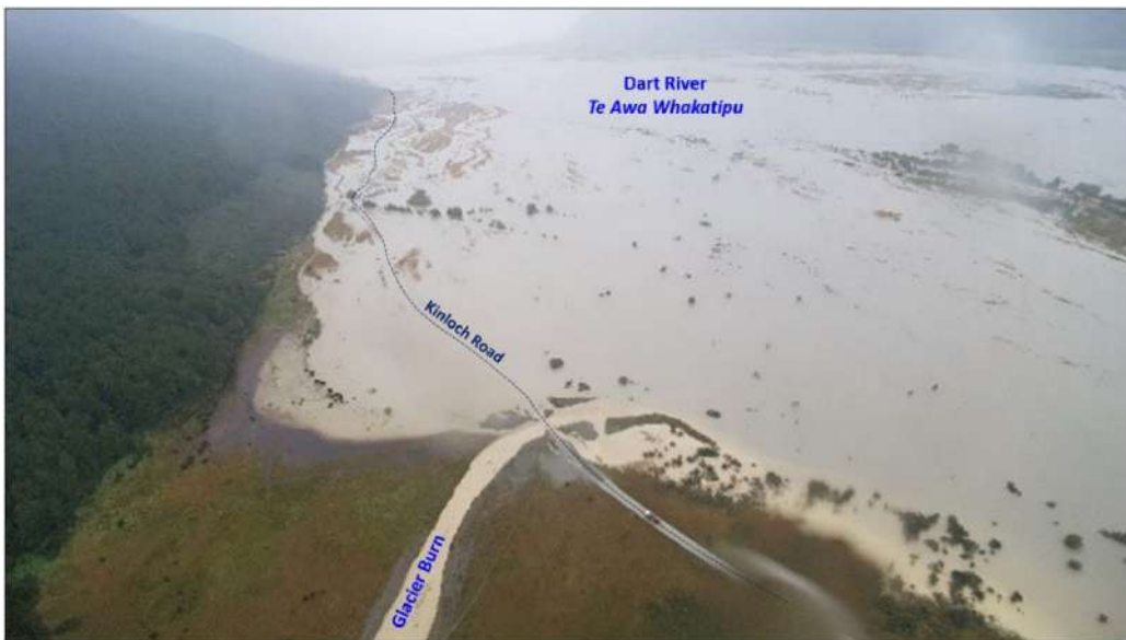
Figure 20: Flooding of Dart floodplain, showing inundation of Kinloch Road (March 2019).
