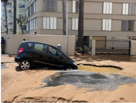
Pipe leakages up to pipes bursting
