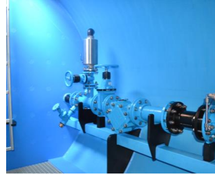
Failure of important fittings in the pipe network
