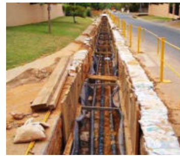
Integrated utility relocation
