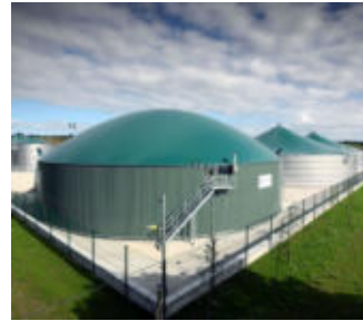
Biogas energy plant
