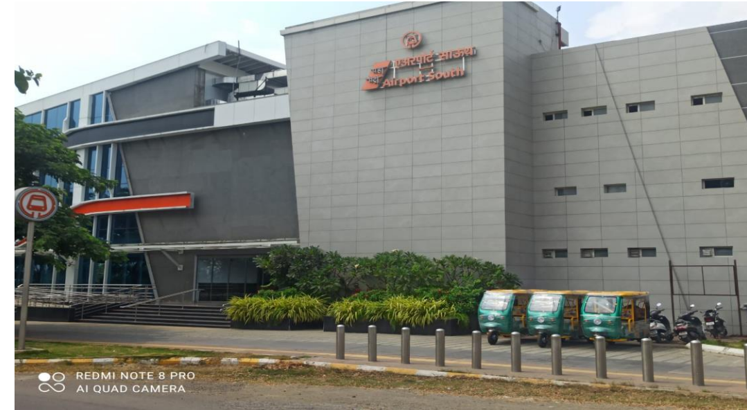
Fleet at Airport South Metro Station
