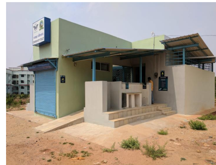
Water & Toilet Service -Cuttack & Bhubneshwar
