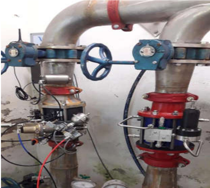
April 2020 – Vertical installation
