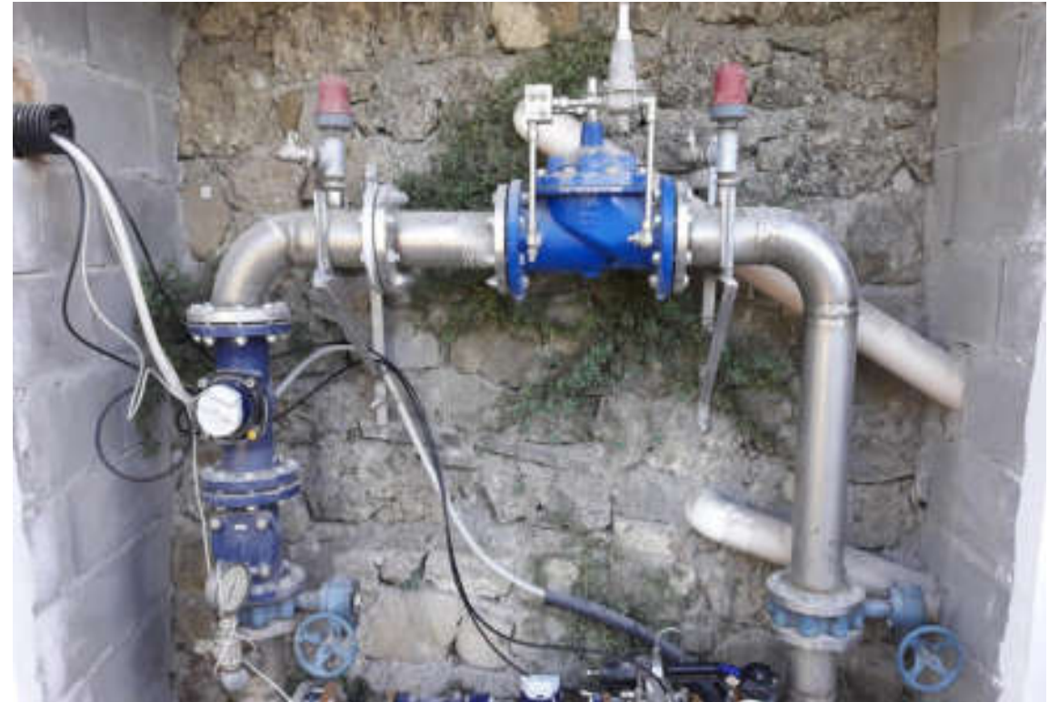
July 2020 – By pass installation
