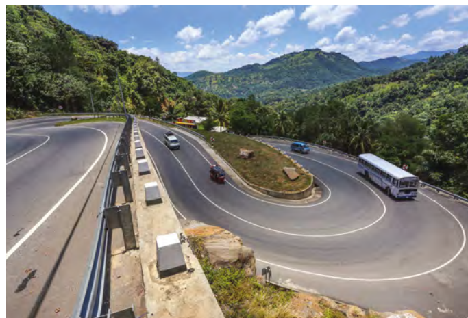
The Kandy-Mahiyangana national highway in central Sri Lanka was upgraded under the ADB-supported National Highways Sector Project.
