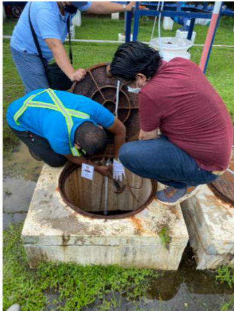
1 Reservoir Level Sensor
