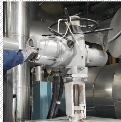
MOTOR OPERATED VALVE
