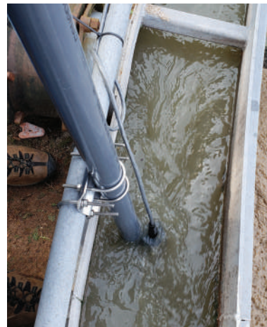
Figure 2.2 Open bio-reactor install
