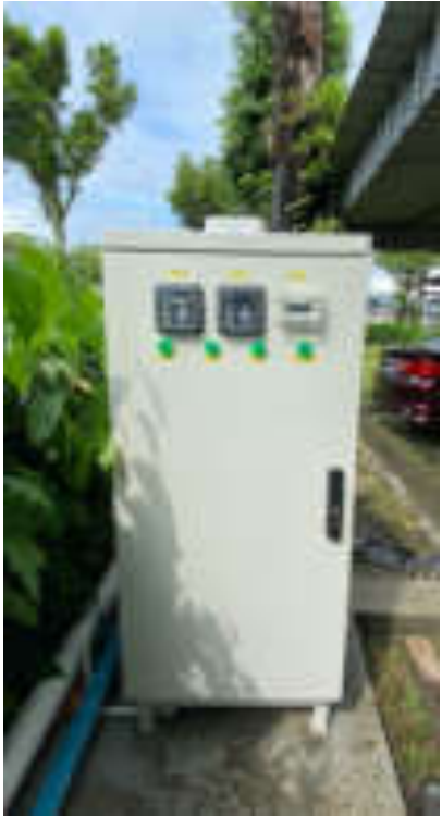
WQ / Illegal Discharge Detection at Factories
