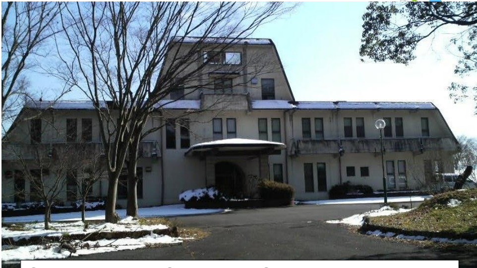
Omihachiman City Night Soil Treatment Plant
