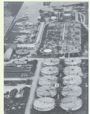
Picture 1 The first large scale night soil treatment plant (Sunamachi plant, capacity 3,600kℓ/day,1954) (6)
