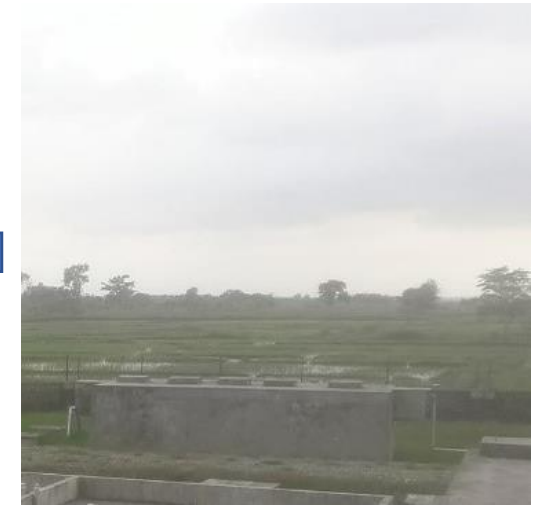
Anaerobic Baffle Reactor
