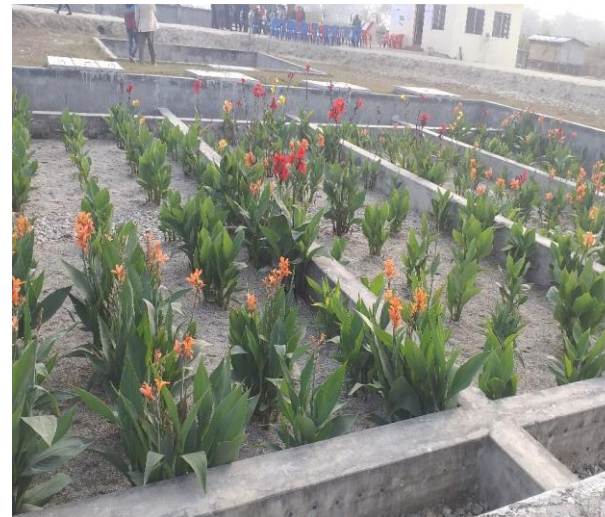
Planted Gravel Filter
