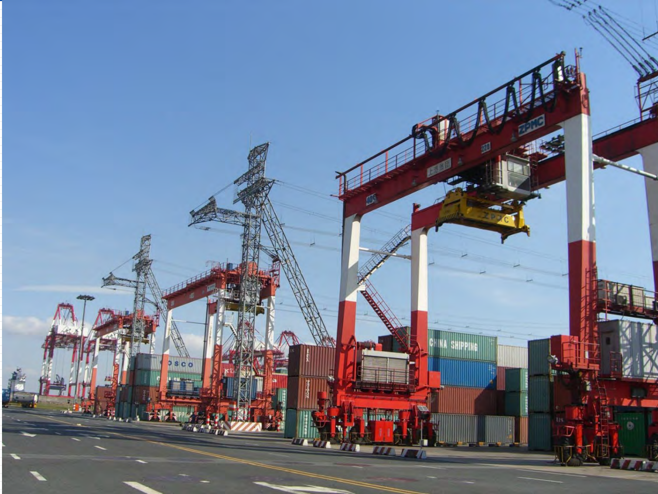
High-altitude container area-crossing isolated conductor rail
