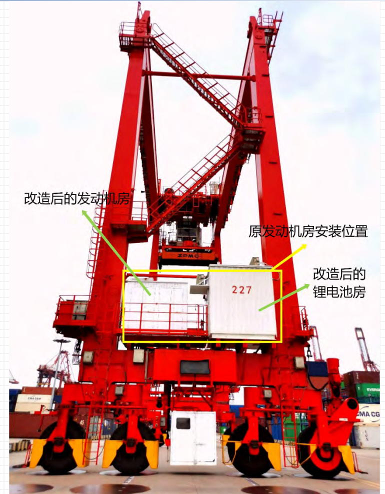
Modification of Lithium Battery Diesel Hybrid Power for Tire Crane
