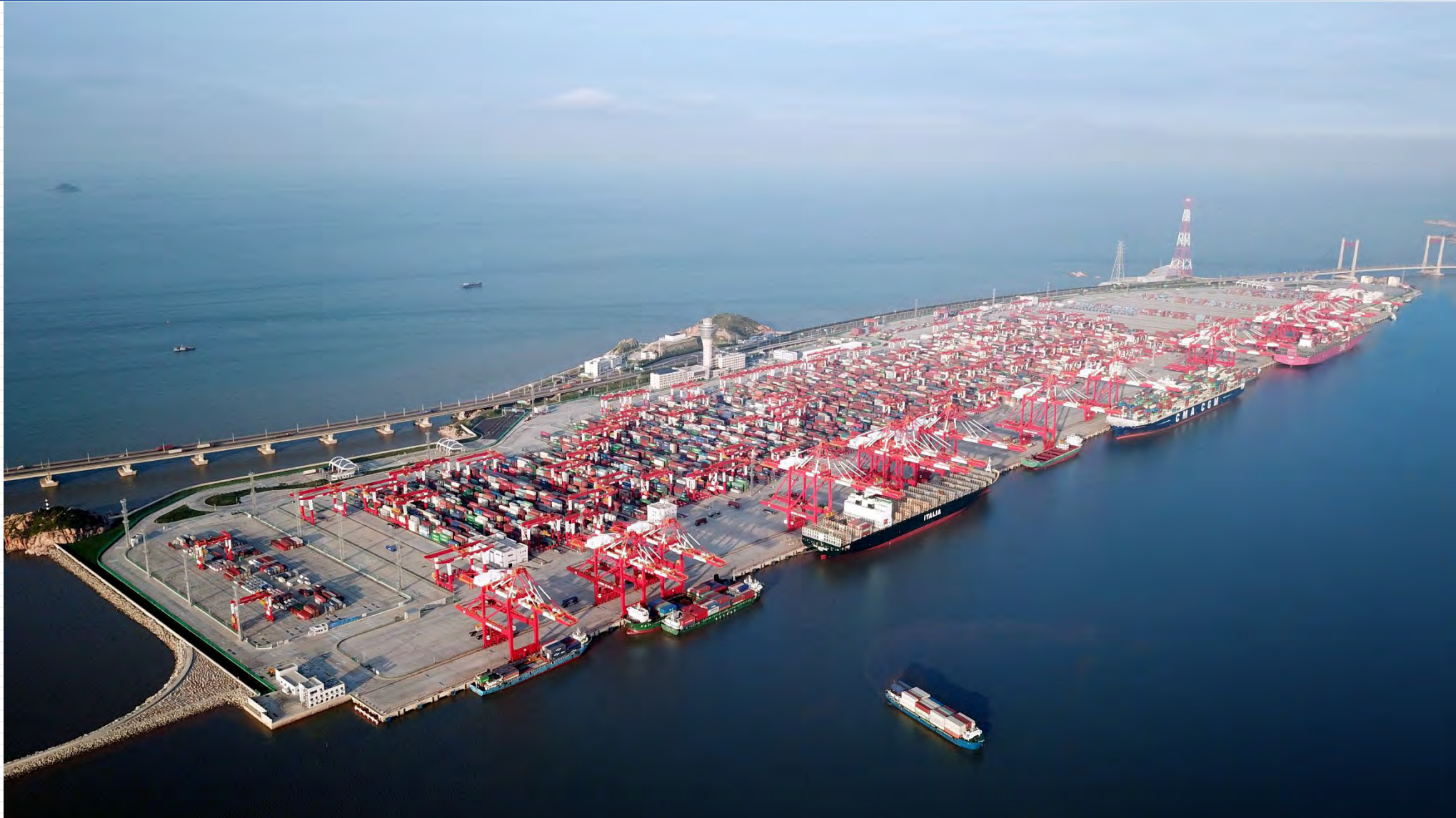
Yangshan Phase IV Fully Automated Port Area-Full Electrification of Loading and Unloading Equipment
