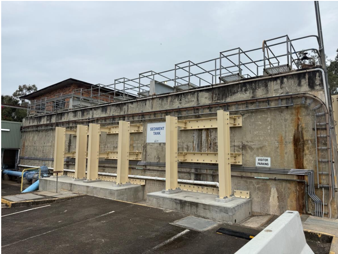
Figure 4 - Sedimentation tank buttressing
