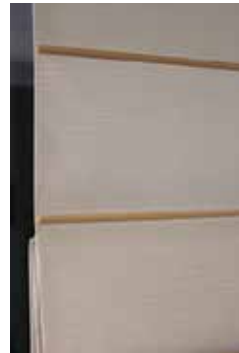
Timber Battens Front
