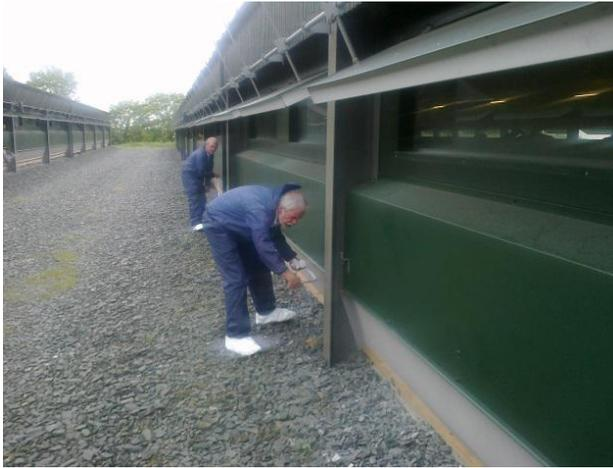
Figure 2 - Flyscreens being attached to the air inlet.
