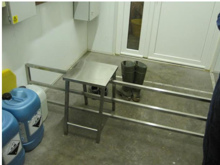
Figure 1 - Hygiene barrier in annex to bird area. (Note other designs are solid to prevent migration of litter material under the barrier).
