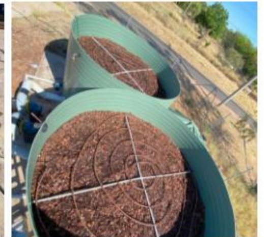
DN50 irrigation pipe with media support at 300mm
