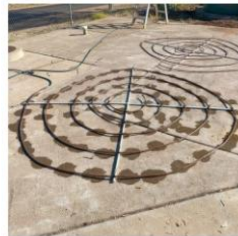
DN50 irrigation pipe with media support at 300mm
