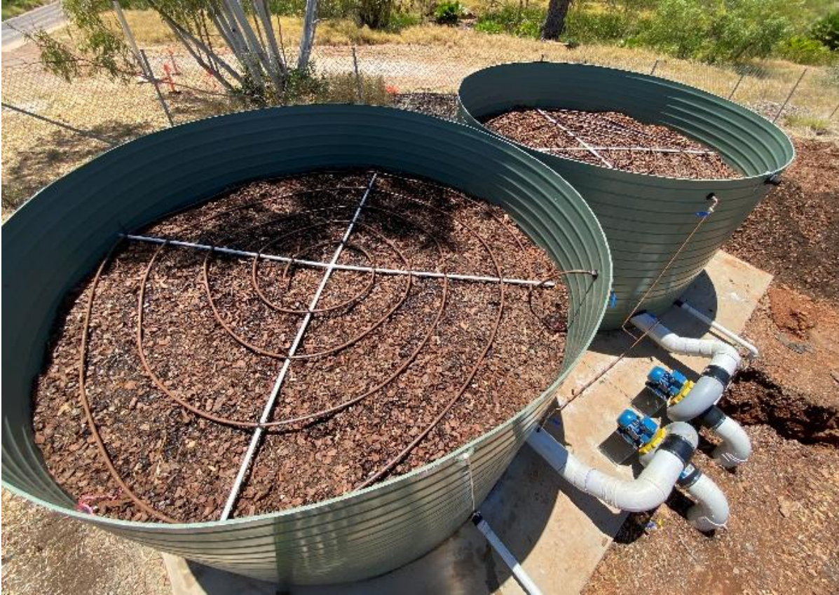
DN50 irrigation pipe with media support at 300mm
