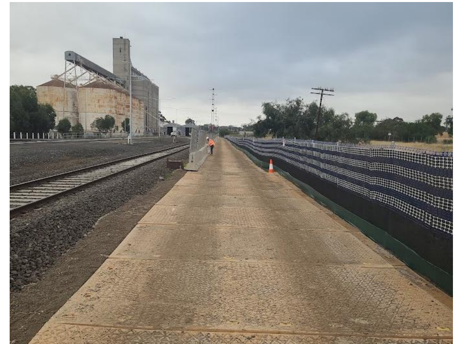
Example: installation of bog mats on unsealed access tracks
