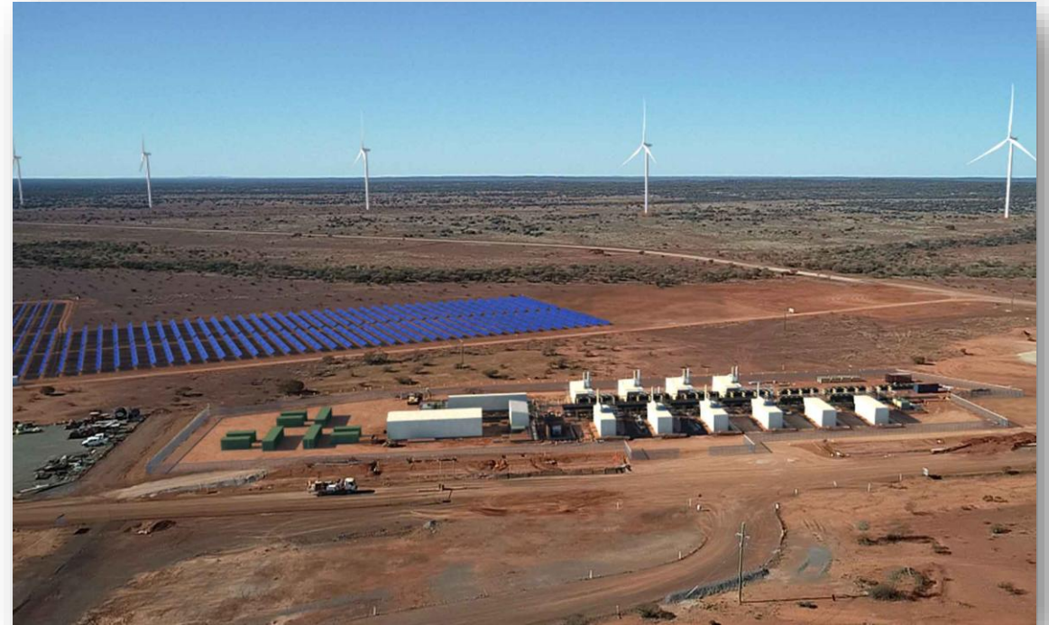
Wind turbines, solar farm and batteries at EDL's Agnew Hybrid Renewable Microgrid site supporting the Agnew Gold Mine (WA)
