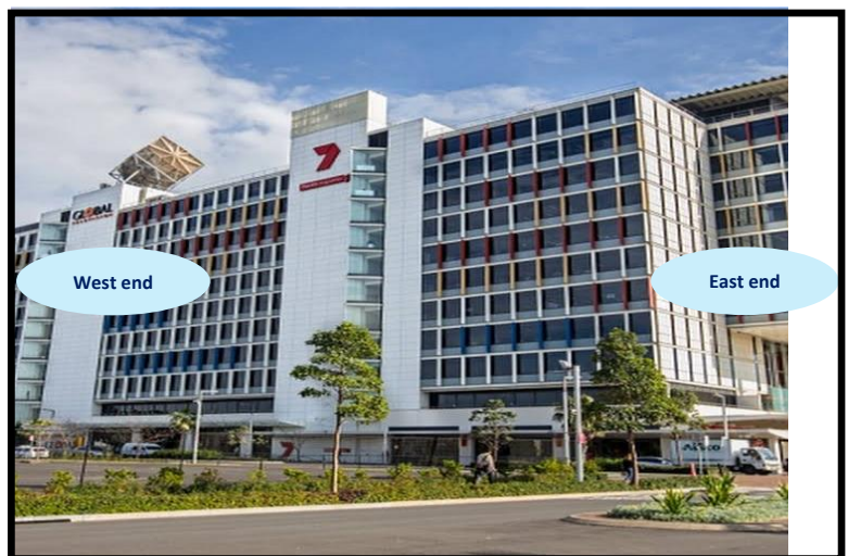
Central Avenue Building
